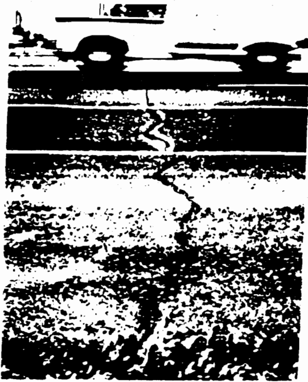
Transverse Cracking
