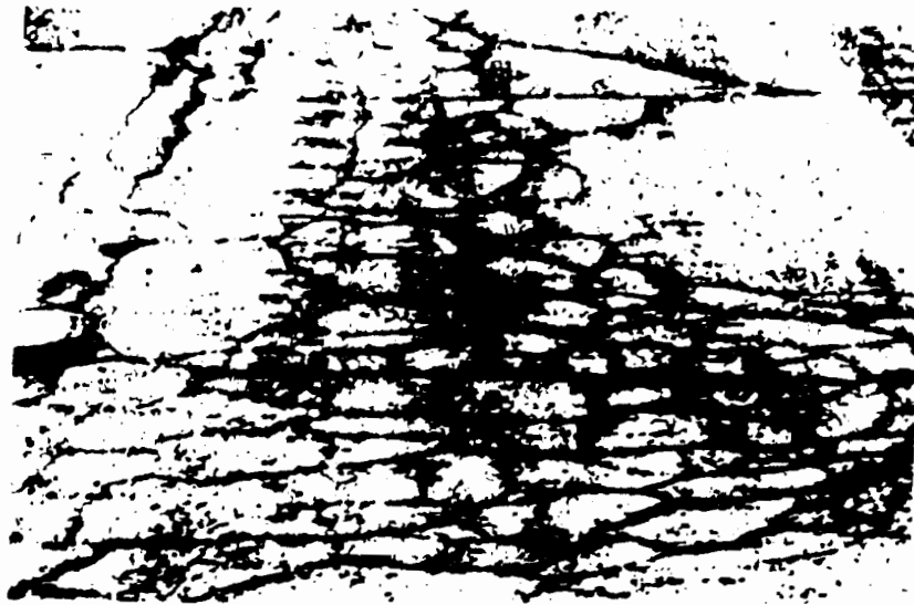
Alligator Cracking
