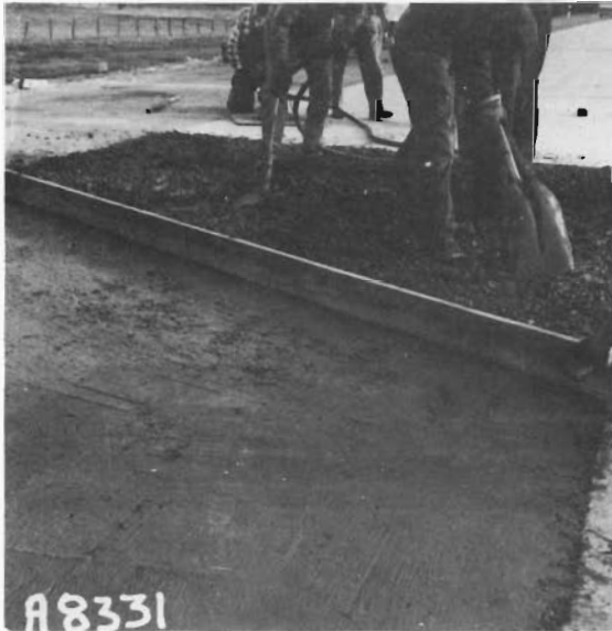
FIGURE 19 Hand finishing and vibration.
