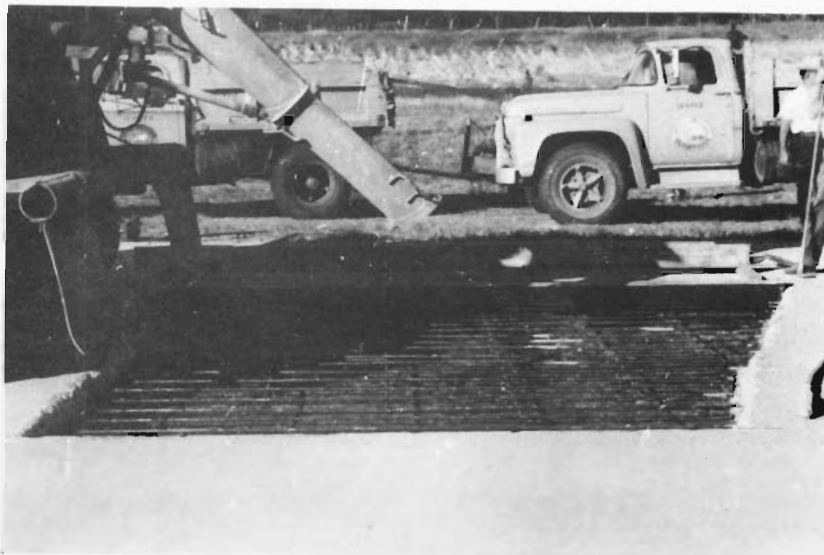
FIGURE 15 Ready for concrete placement.
