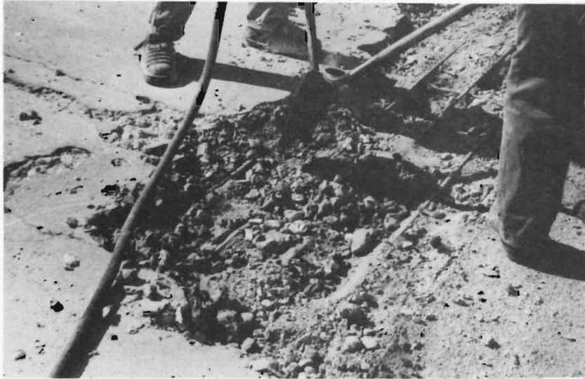
FIGURE 5 Jackhammer breaking concrete which is being removed by hand method.
