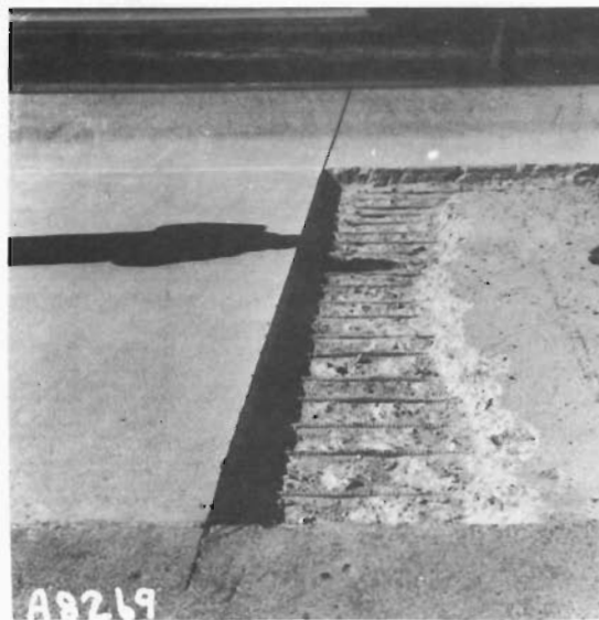
FIGURE 10 Concrete removed from steel to be left for lapping to new steel.
