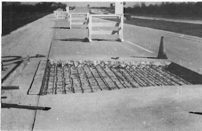
FIGURE 14 Exposed faces of pavement slab painted with epoxy bonding agent.
