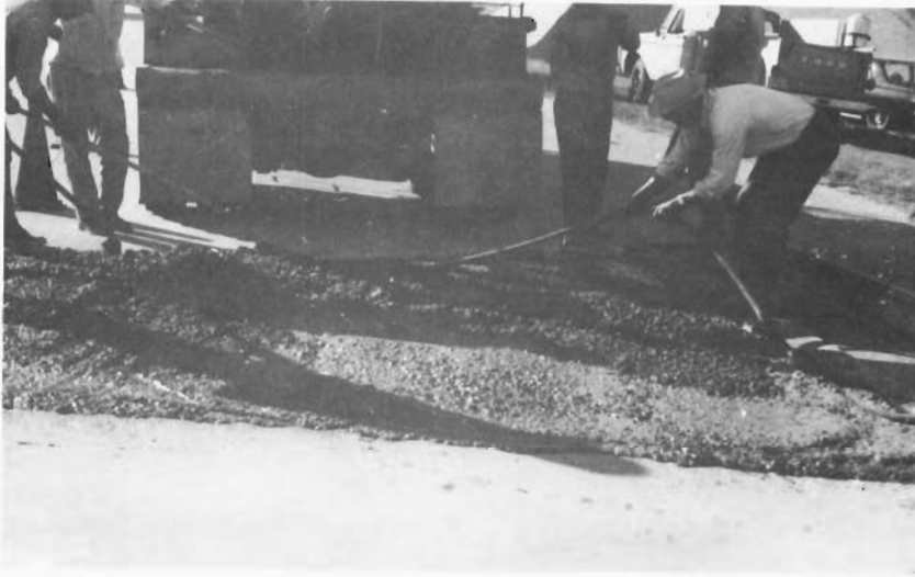
FIGURE 17 Vibrating concrete with hand manipulated vibrator.
