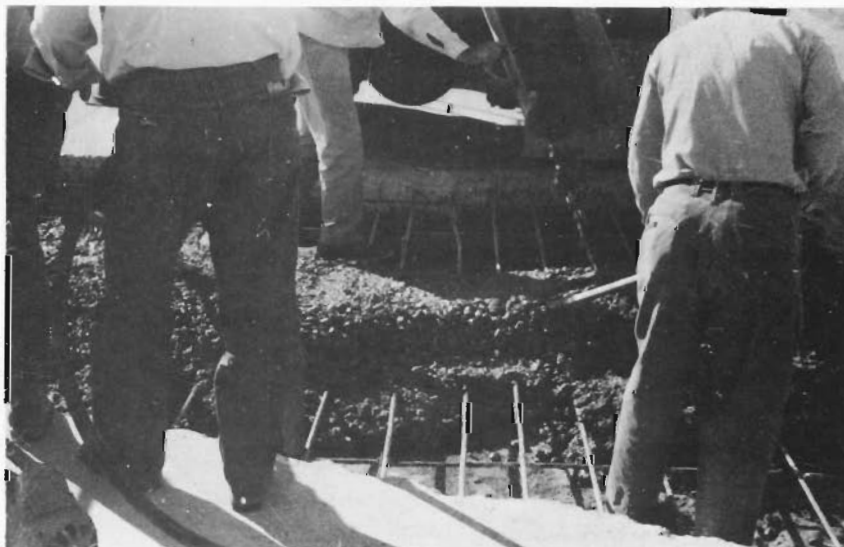
FIGURE 16 Concrete being replaced in repair area.
