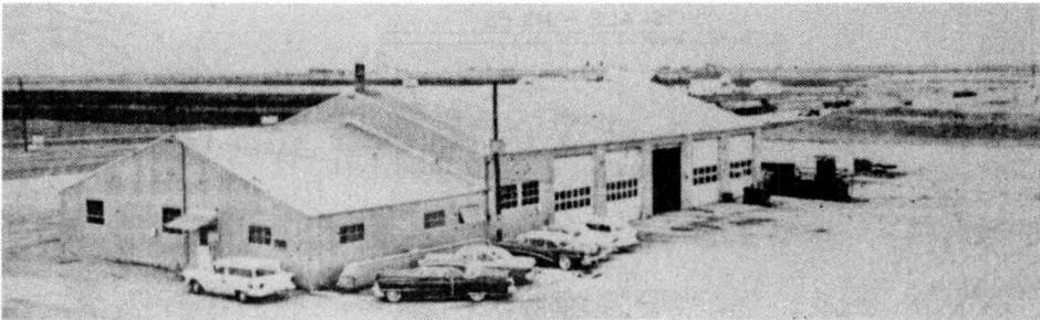
Figure 5. Vehicle maintenance garage.
