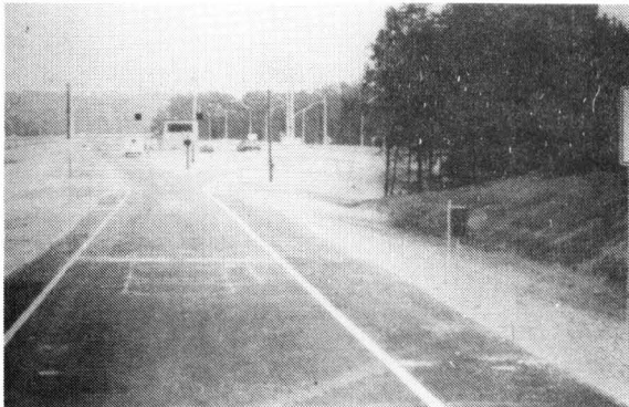
Slide 9.14. Installation of WIM system.
