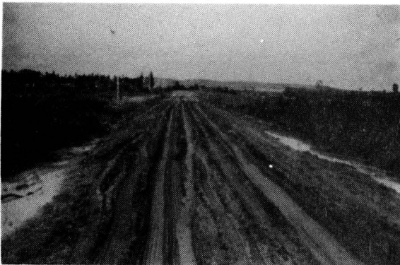
Slide 4.5. Unpaved roads should also be considered in a PMS.
