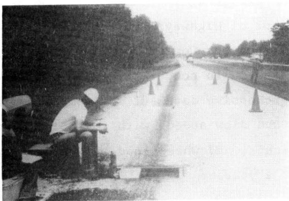
Slide 9.3. Arrangement of traffic control.
