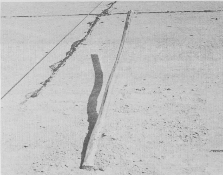
Figure 9. "Before" and "After" photographs of Mile Post Marker mounted on 1.25" pipe embedded in 8" diam. concrete shaft. Test S-12, 56.9 mph.
