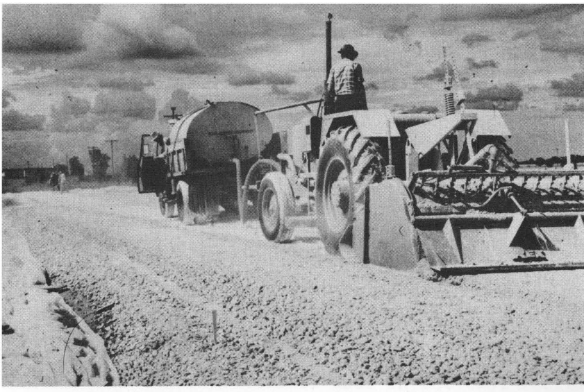
Figure 3: Test facility construction. Spreading crushed limestone (upper) and mixing water and lime with Rex Chain-Belt Pulvimixer (lower)
