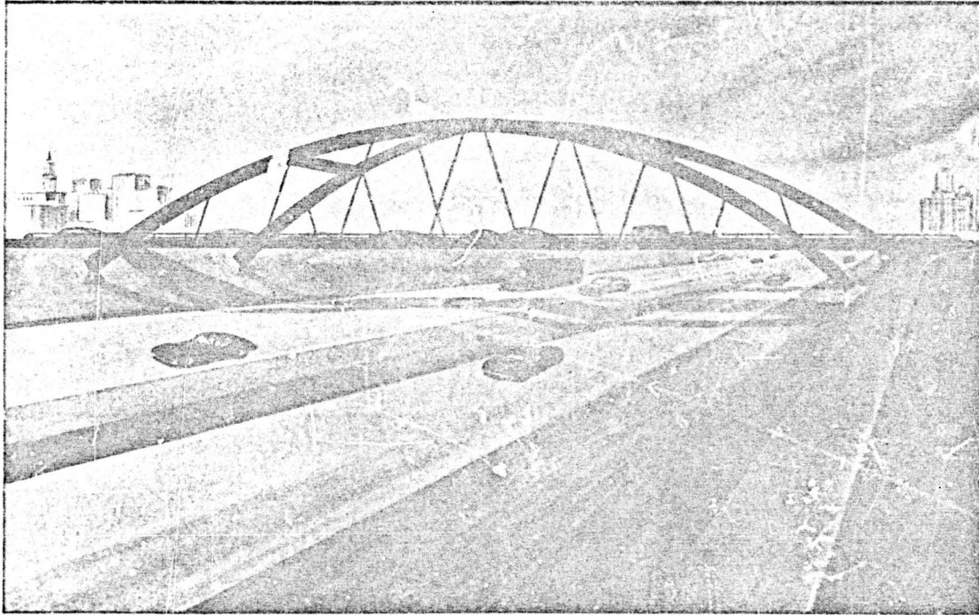
FIGURE 2. ARTIST'S SKETCH OF LEANING ARCHES BRIDGE CONCEPT IN NEW BRIDGE APPLICATION
