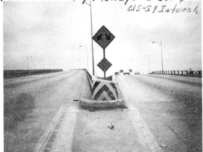
Figure 11. Typical Hazardous Locations Where Barrel Protective Barriers Could be Employed
