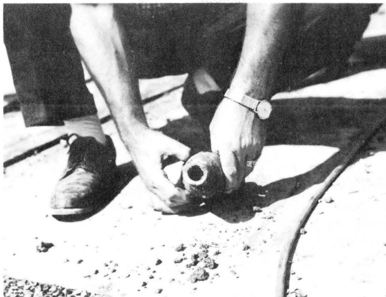
Figure 20, Connection From Which Cable Pulled Free.
