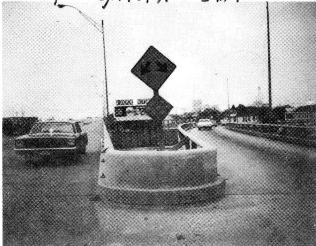
Figure 11. Typical Hazardous Locations Where Barrel Protective Barriers Could be Employed
