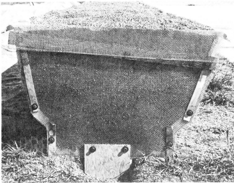
Figure 3 , End View of Fiberglass Median Barrier
