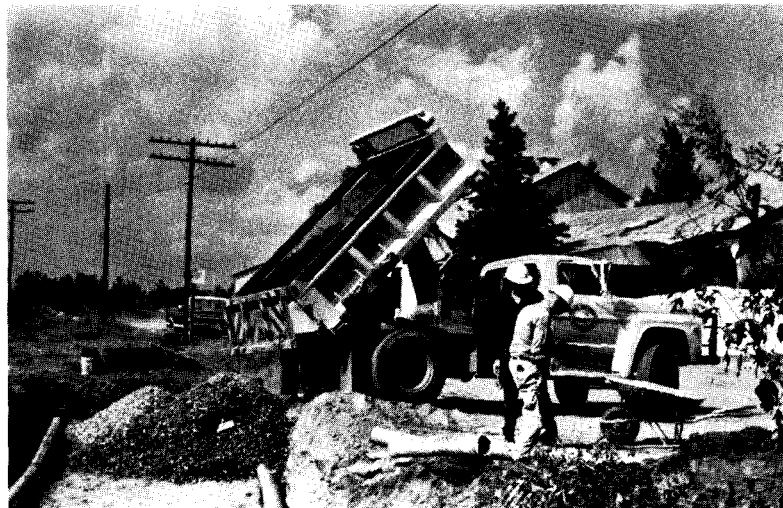
FIGURE 3-4 - LIMESTONE BALLAST COVERING SUBDRAIN PIPES
