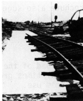
REPLACING TRACK STRUCTURE
