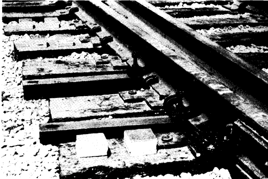
FIGURE 2-7 - SHIMS AND HARDWARE FOR FAB-RA-CAST SLAB
