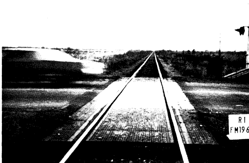
FIGURE 2-2 - RUBBER PANEL CROSSING INSTALLATION AT FM HIGHWAY 1960 AND ROCK ISLAND RAILROAD
