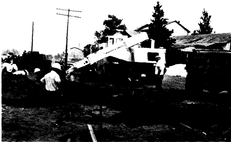
FIGURE 3-1 - BACKHOE LEVELING BASE MATERIAL
