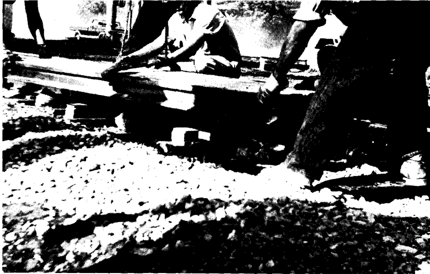
FIGURE 2-5 - PLACING A FAB-RA-CAST SLAB ON GROUT-FILLED BAGS
