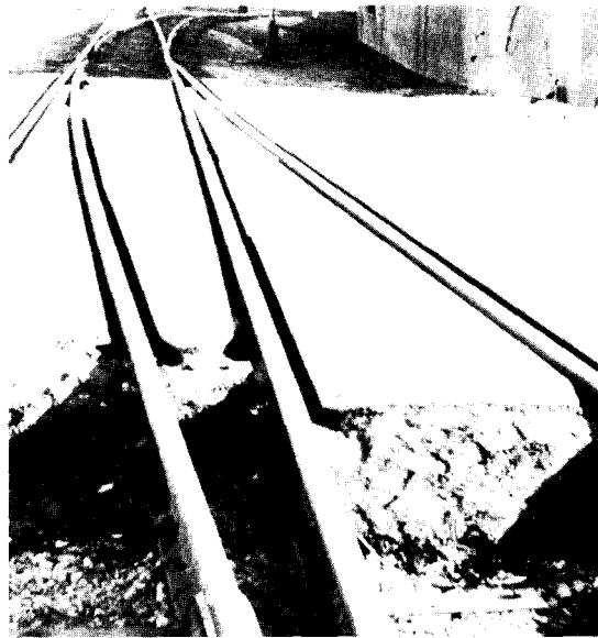
FIGURE 2-9- A COMPLETED FAB-RA-CAST CROSSING WITH A TURNOUT
