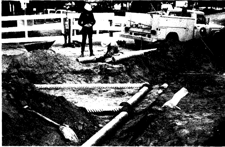
FIGURE 3-3 - OUTFALL LINE FOR SUBDRAIN SYSTEM
