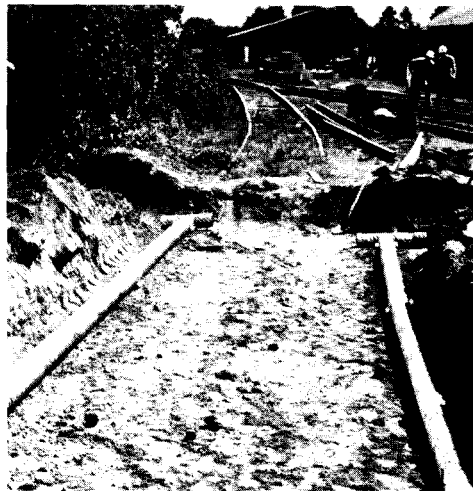
FIGURE 3-2 – TWO STRINGS OF PERFORATED SUBDRAIN PIPE
