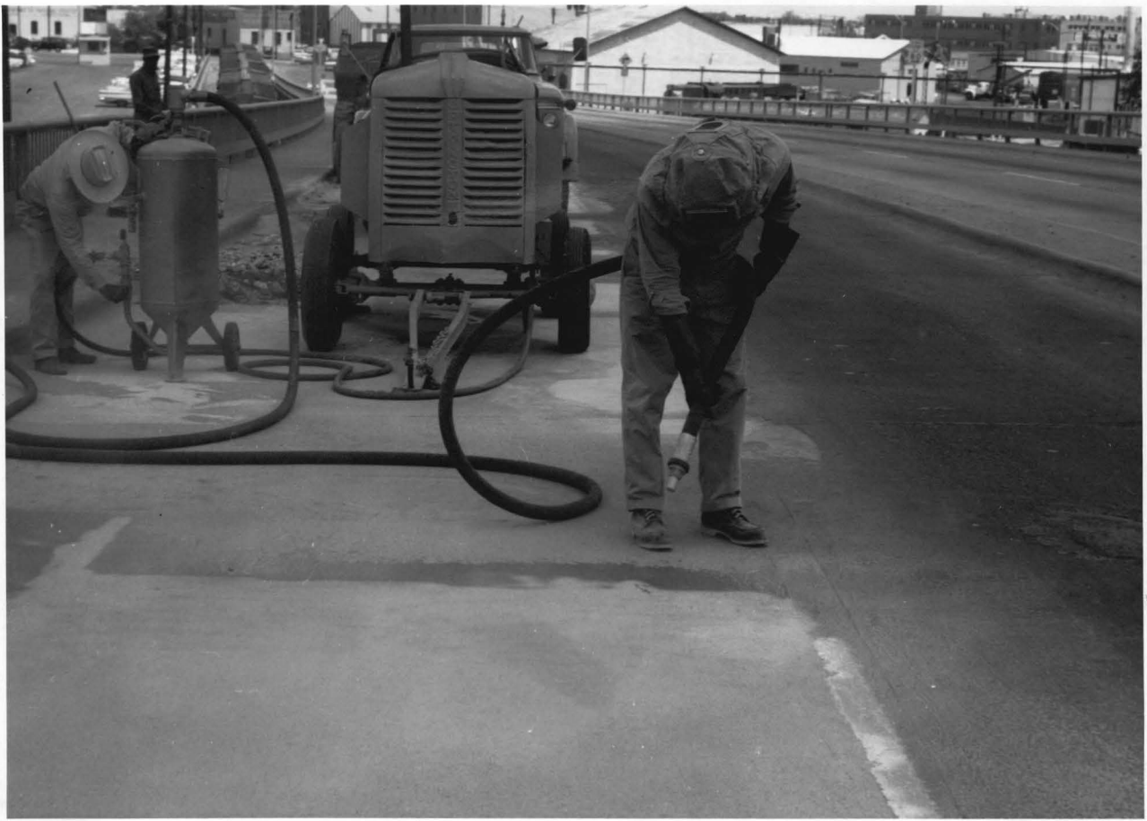
Velasco turns on the air and Aguirre operates the nozzle preparing the deck to receive a Guardkote epoxy seal.
