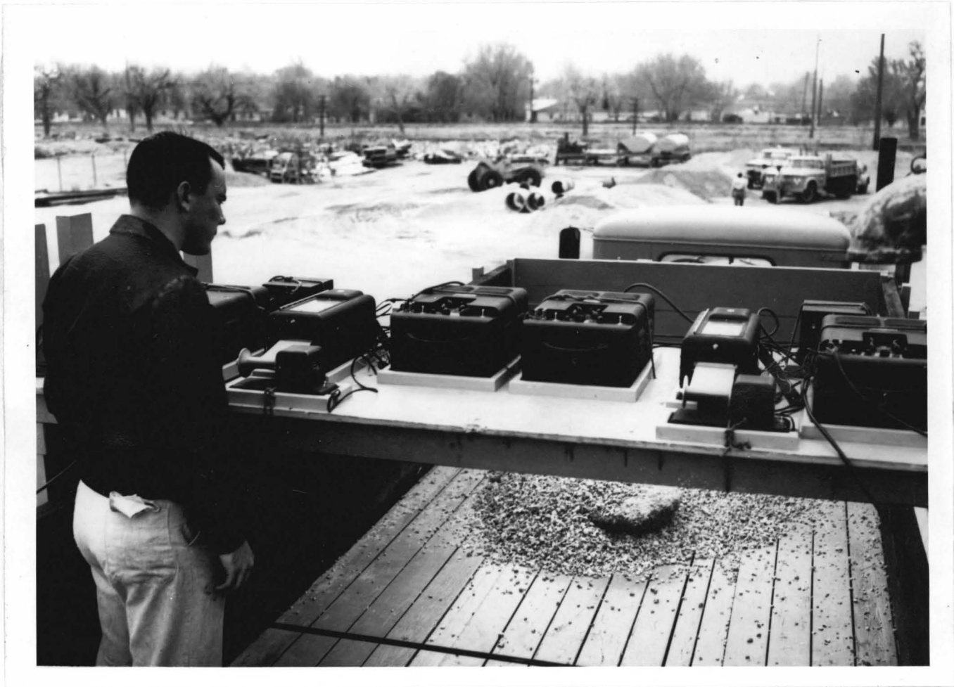
Ed Payne of District Bridge Division calibrates truck mounted instruments as Bureau of Public Roads' test truck is loaded.
