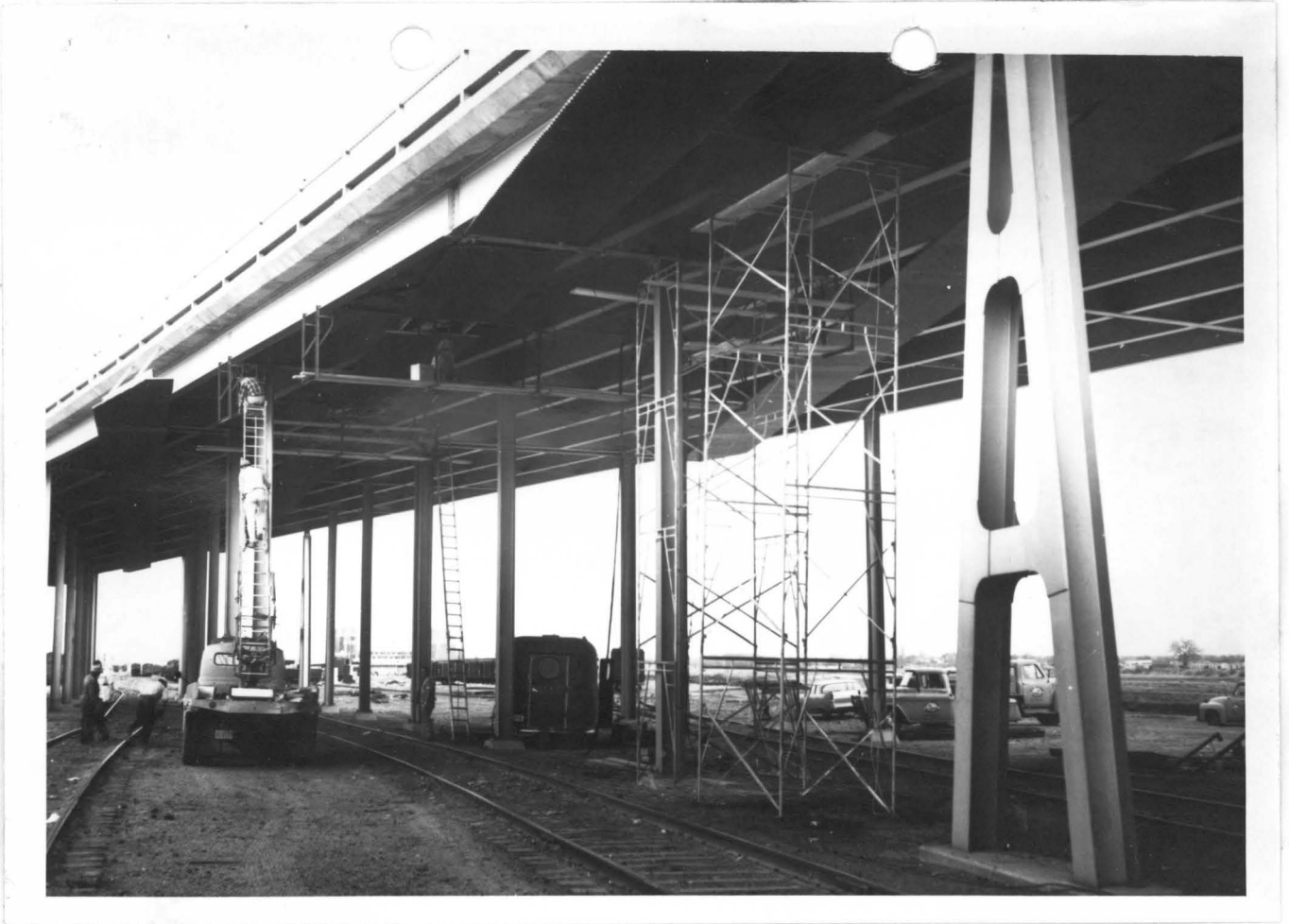
Strain and deflection gauges being placed. Bureau of Public Roads instrument trailer in center. Old Mexico on right.
