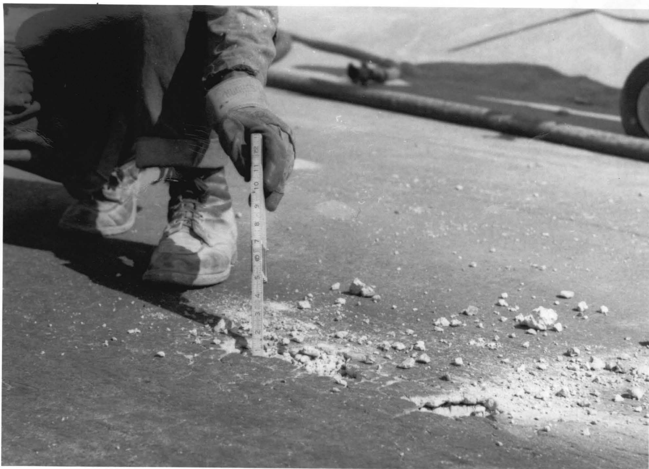
Typical View of Pothole Development
