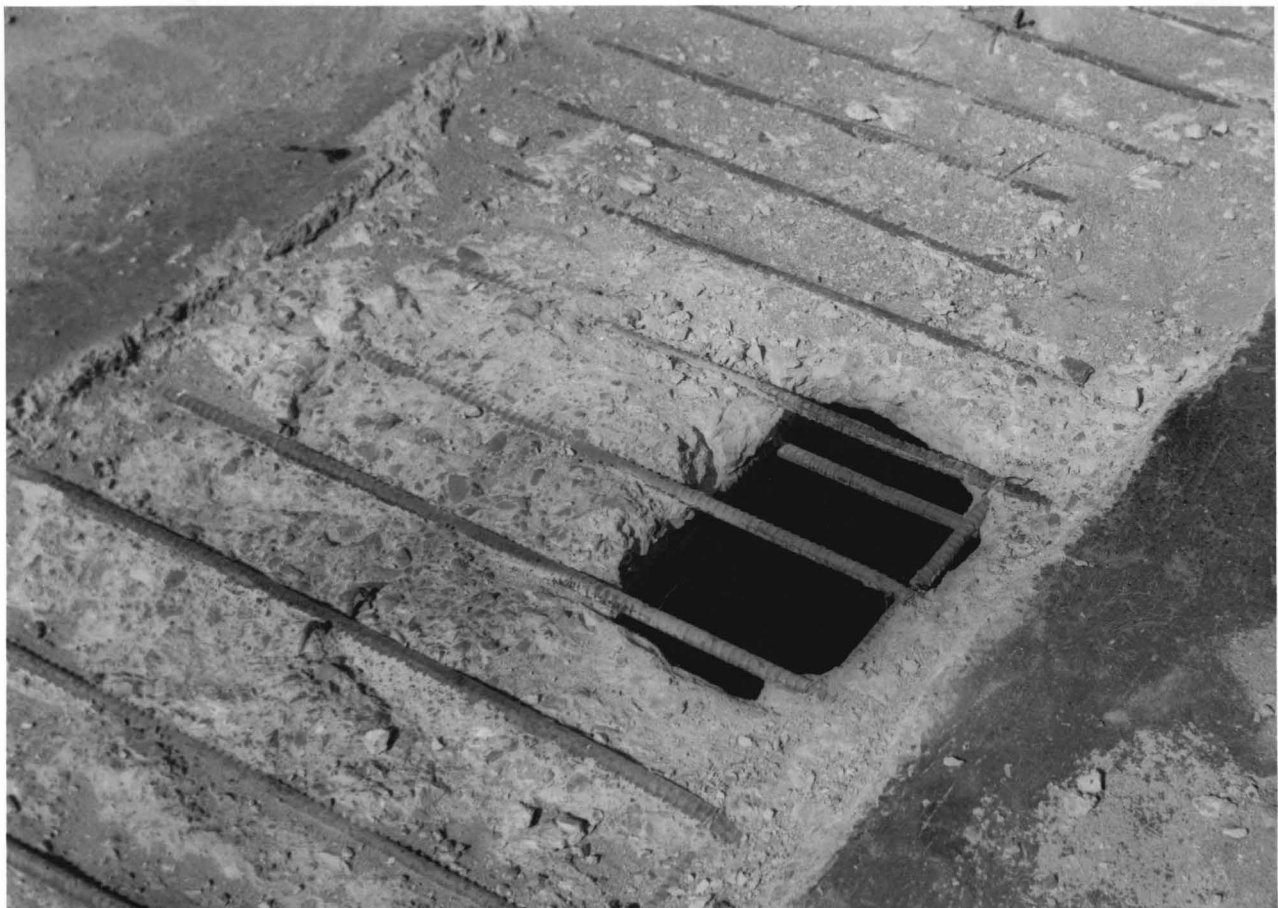
One of three holes opened in deck during operation
