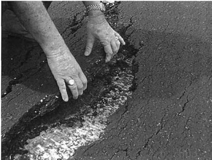
Figure 2.1 - Separation of Overlay Layer Due to Poor Bonding on US-17 in Florida
