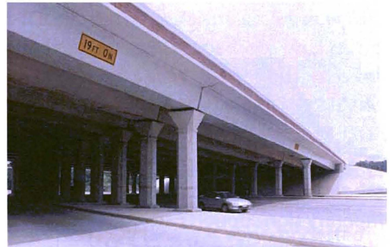
High Strength Concrete girders, Louetta Road overpass structure at US 59, Houston.
