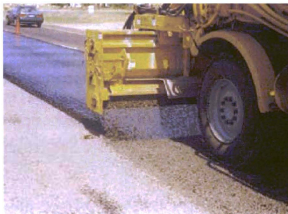
Application of aggregate during seal coat construction
