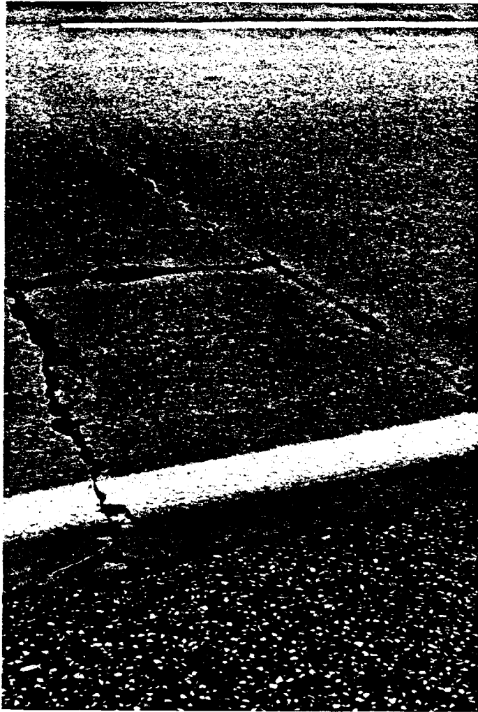
Figure 5.- Severe Punchout
