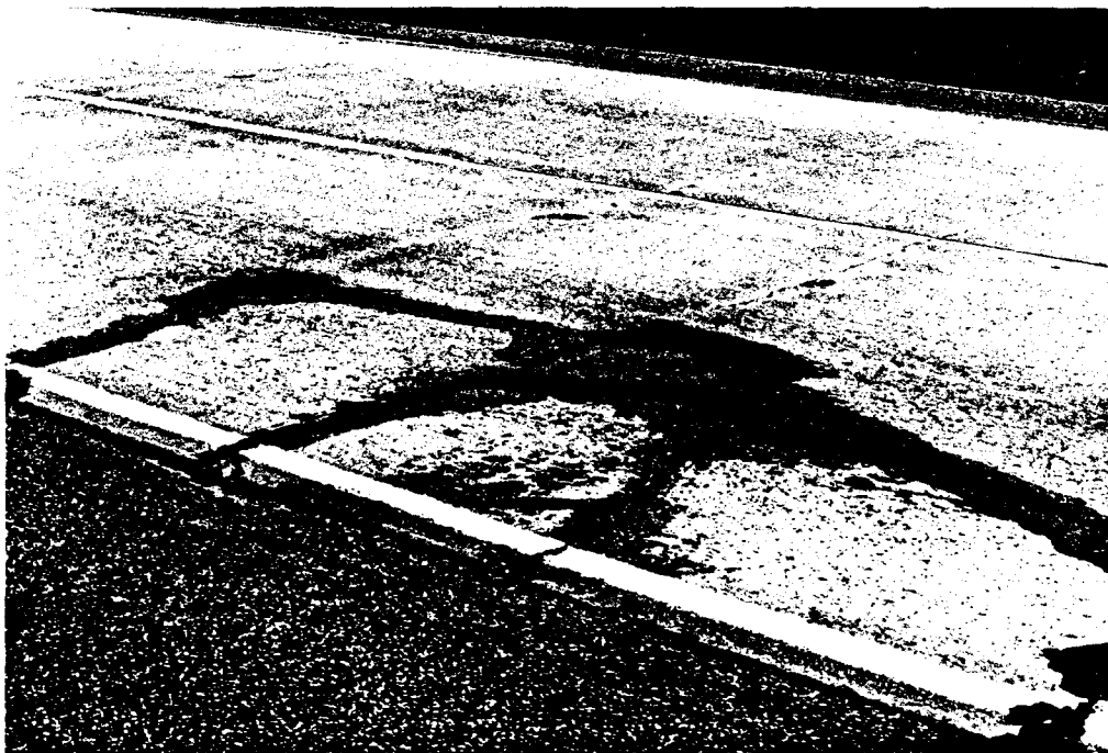
Figure 6. Multiple Punchouts in CRCP
