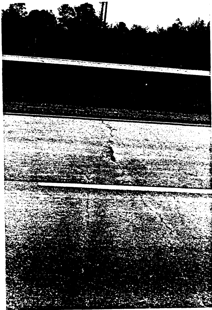
Figure 4. Y-cracking in CRCP
