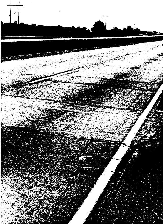
Figure 7. Typical PCC repair patches in CRCP
