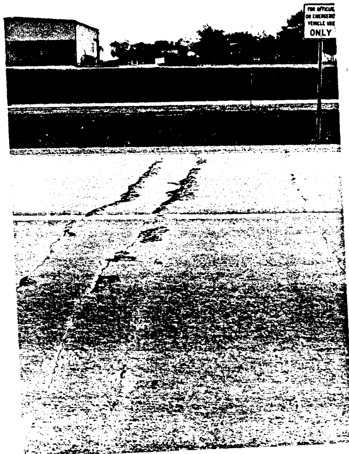
Figure 2. Closely spaced severely Spalled Cracks.
