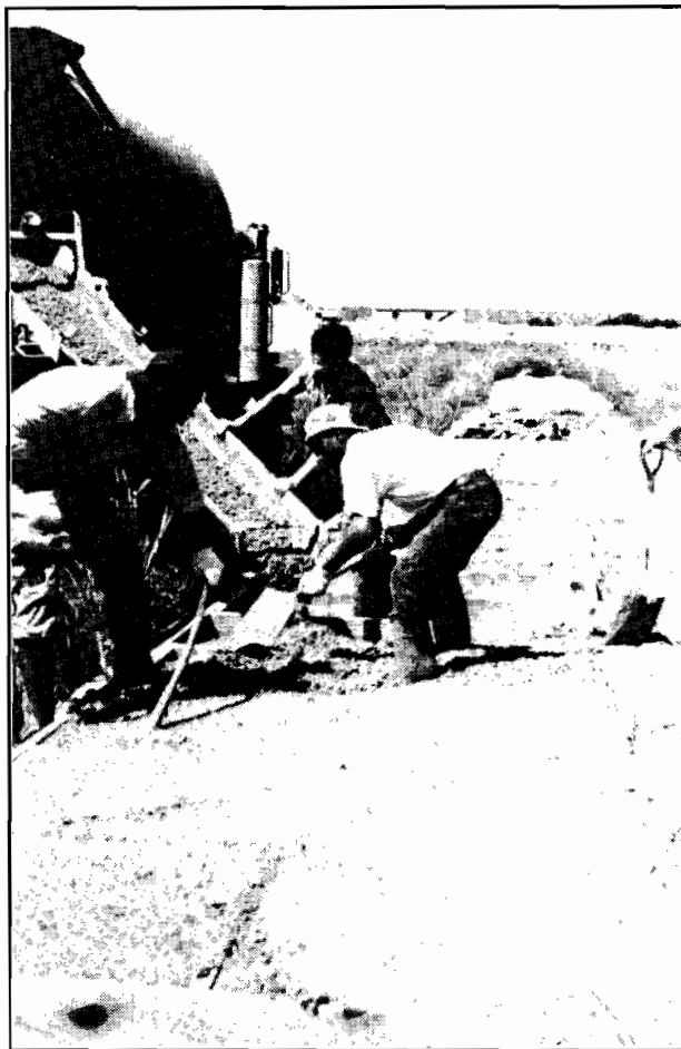
Figure 3.1 Slab specimens for laboratory study are made in large gang forms
