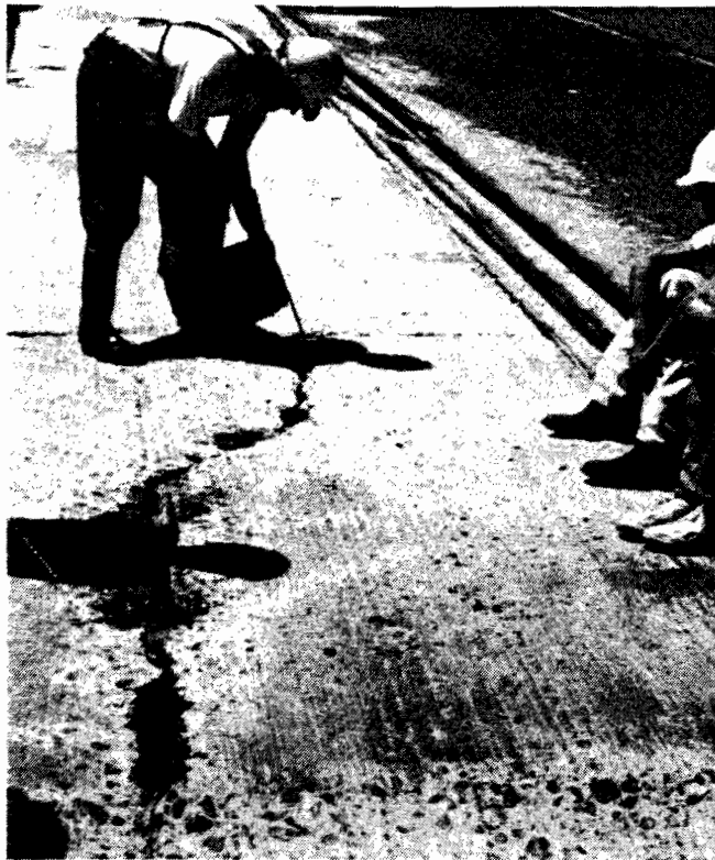
Fig 2.6. Application of monomer.
