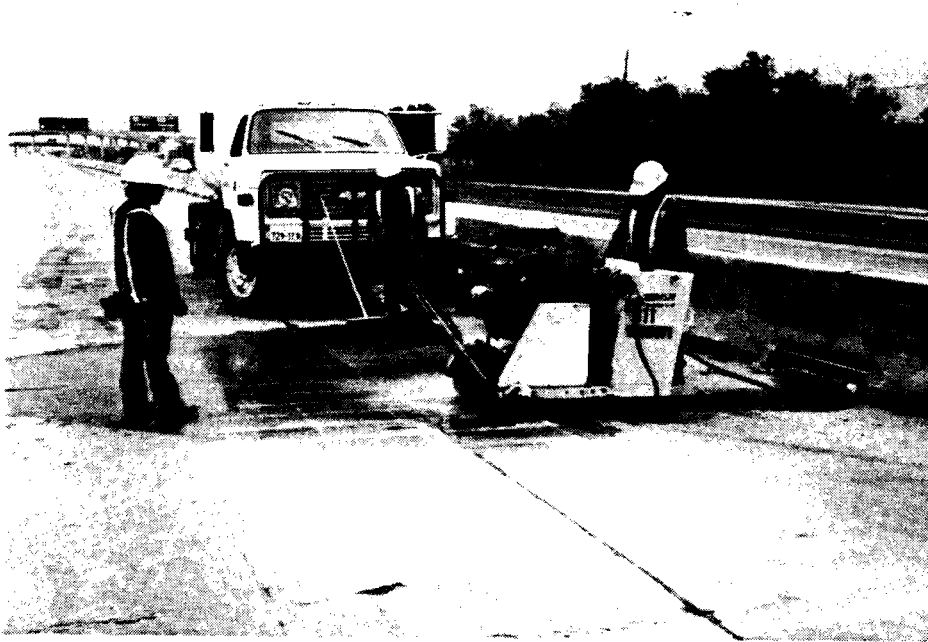
Fig 3.2. Stitching repair process - cutting slots.
