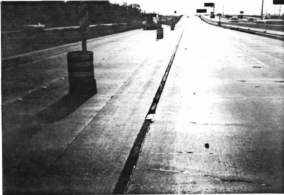
Fig 1.2. Failed longitudinal joint.
