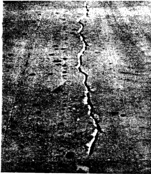
Fig 2.4. Routed crack.
