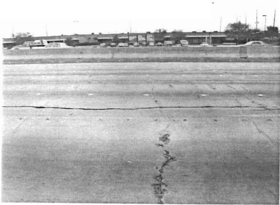
Fig 1.4. Spalling.
