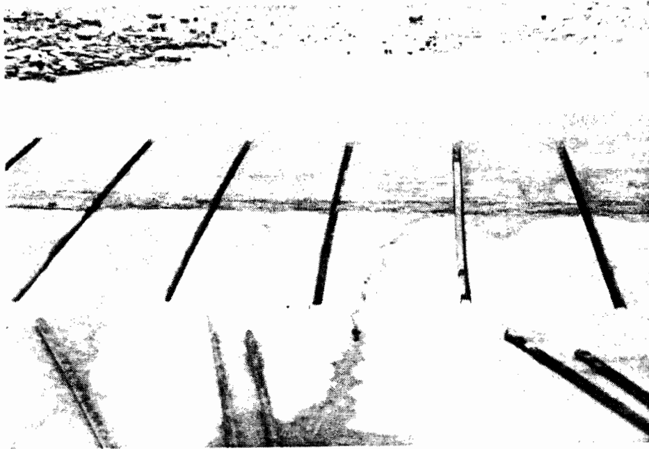
Fig 3.3. Stitching repair process—bar placement.
