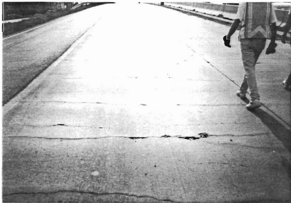
Fig 1.3. Transverse cracking.
