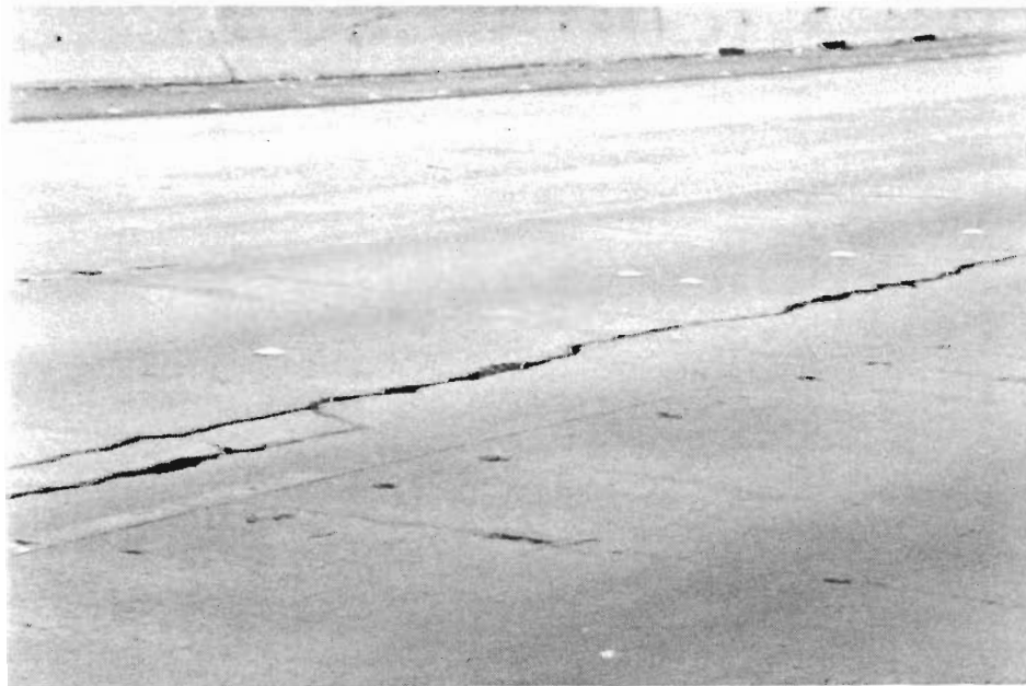
Fig 1.1. Uncontrolled longitudinal cracking.
