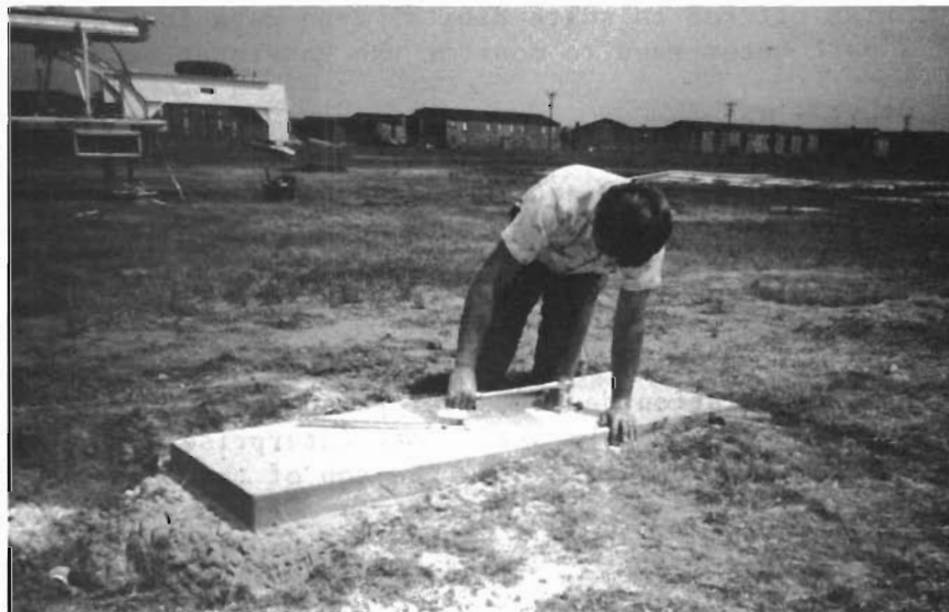
Figure 2 - SWECS Foundation
