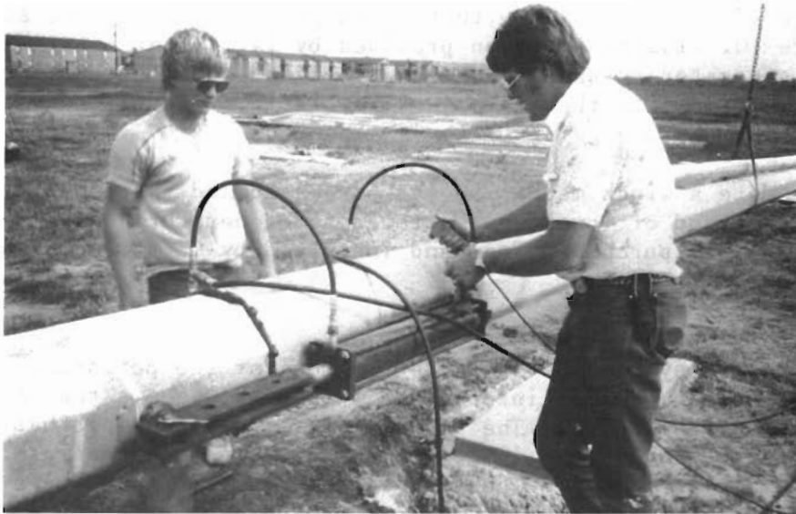
Figure 4 - Connection of Tower Lengths
