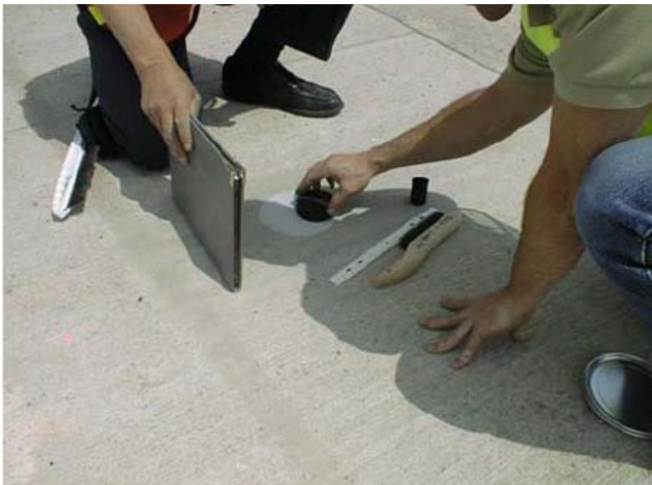
Figure 2-1 Sand patch testing
