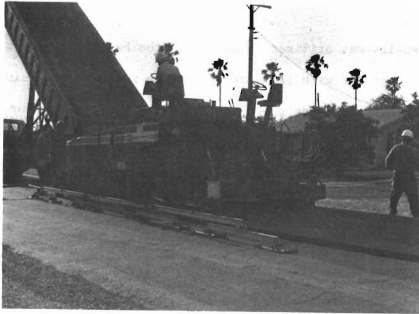
Figure 50. May 7, 1976. Lay down of HMA using flux oil (6:40 p.m.).
