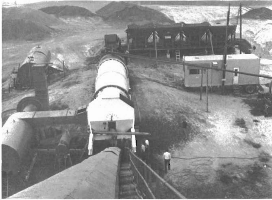
Figure 23. Overview from top of the hot-mixed storage bin.
