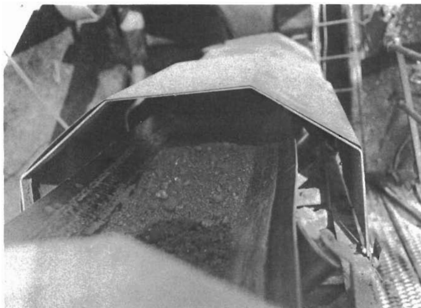
Figure 46. Some large aggregate was processed through. The plus 1-1/2" coarse aggregate was not screened out. This large material caused problems in the laydown phase.
