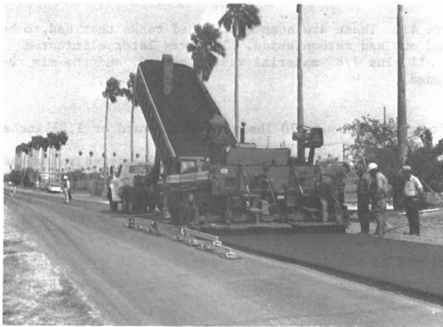
Figure 40. The electronic control rides on a guidewire between two points which multiply down to eight sliding shoes. This smooths out the rough spots of the old pavement.
