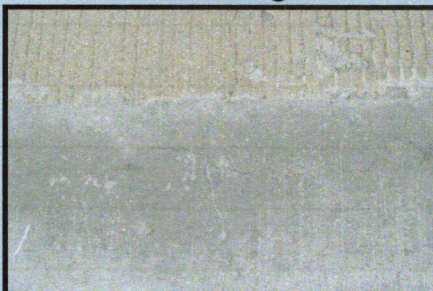
EucoSpeed- note reflective cracking
