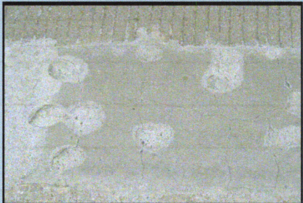
MgKrete- note blisters and cracks
