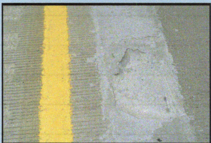
MgKrete- severe spalling
