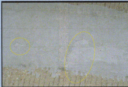
Pavemend- surface spalling
