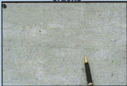
Pavemend—closely spaced cracks
