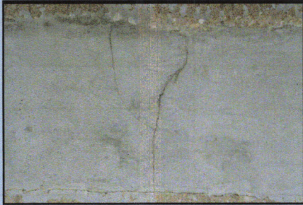
Pavemend- severe cracking
