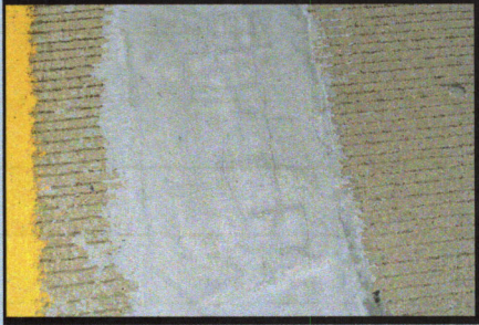
Pavemend- note cracking
