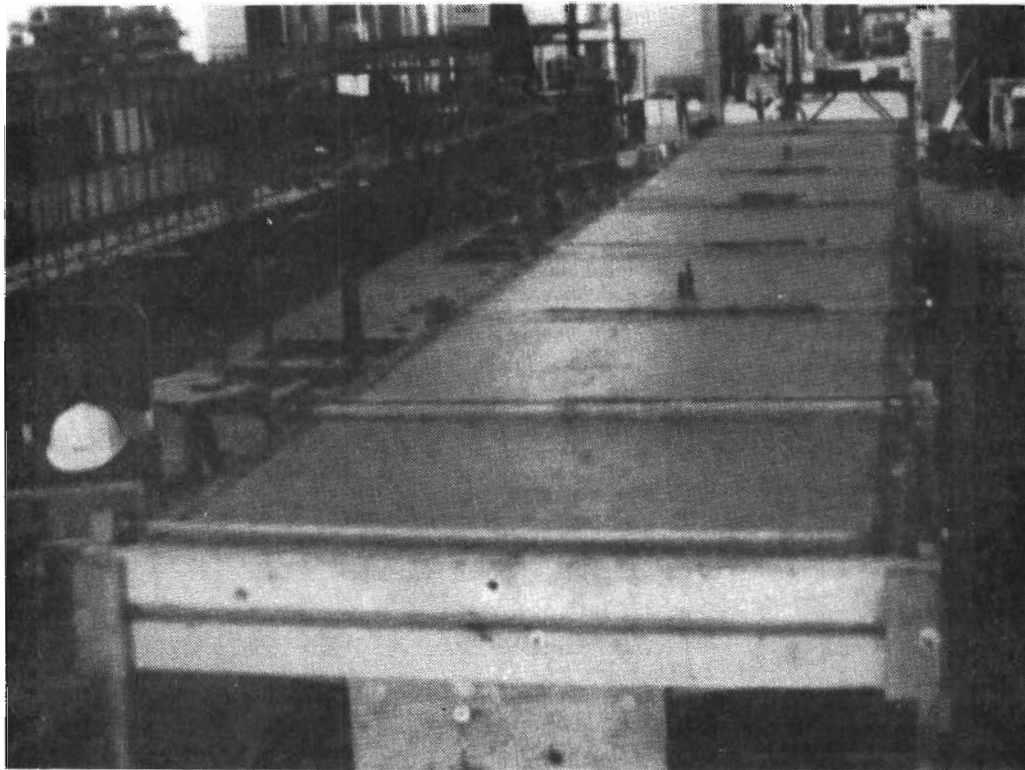
Fig. 2.19 Formwork prior to and after casting
