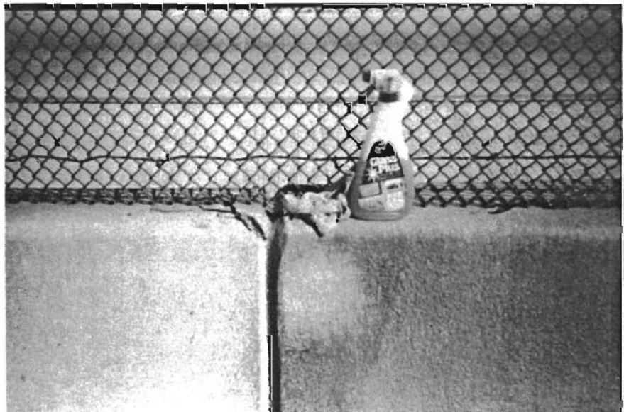
Fig 3.1. Discoloration on median barrier at the Fratt Interchange.
