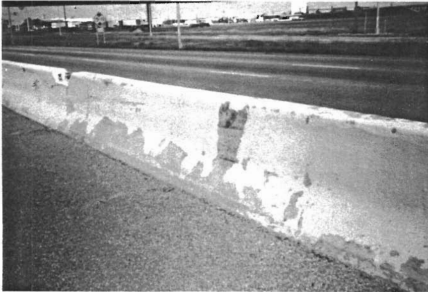
Fig 3.12. Peeling on median barrier in Amarillo.
