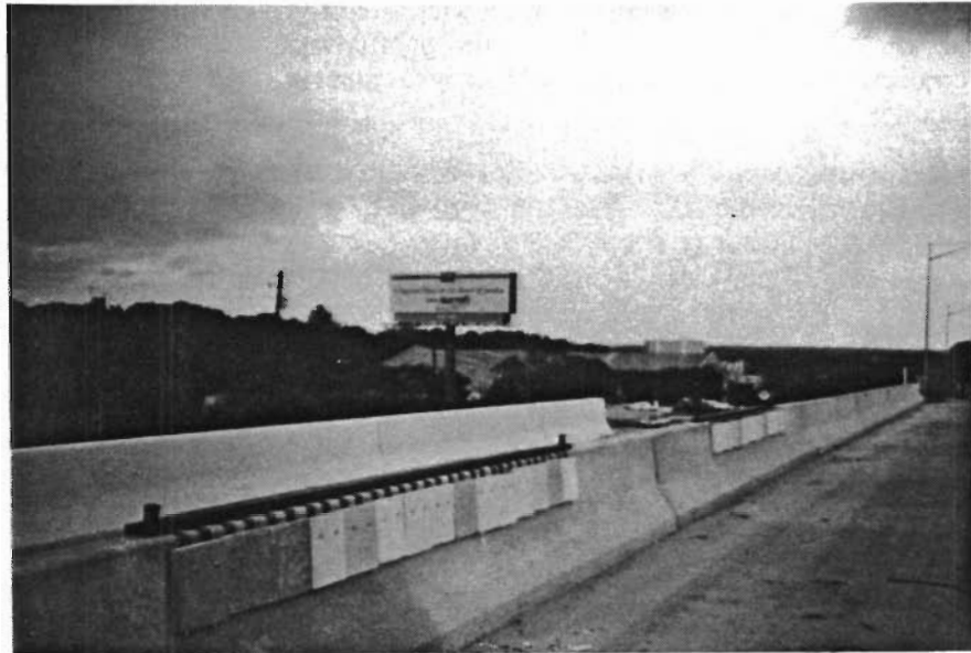
Fig 4.2. Panels in high traffic environment.
