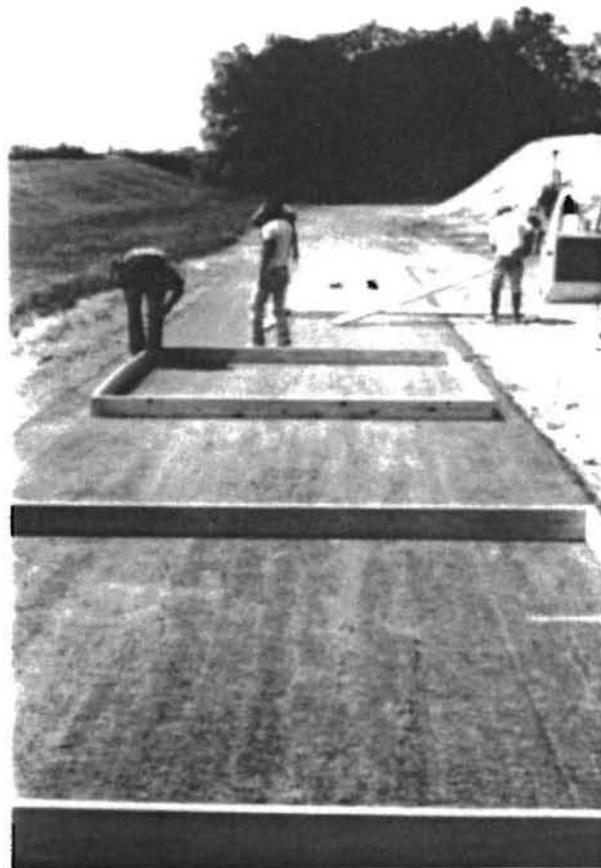
Fig 2.6. Preparation of formwork for slabs.
