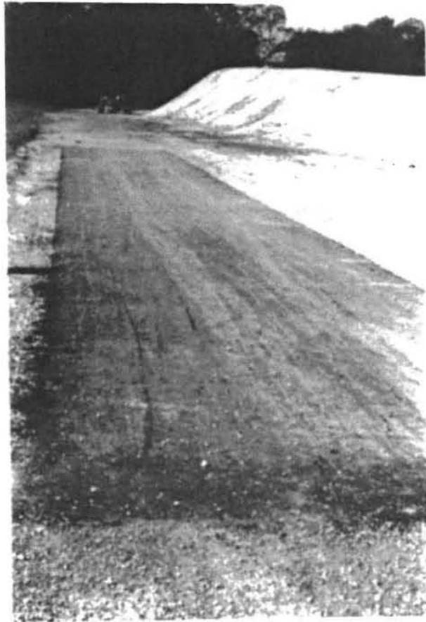
Fig 2.5. Sand mix asphalt pad prepared to provide a smooth surface for the test slabs.
