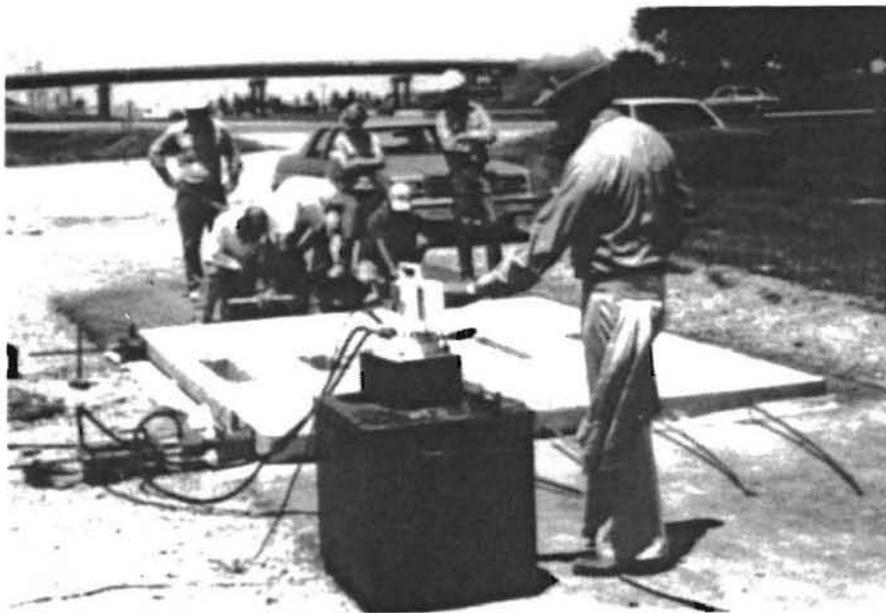
Fig 2.12. Post-tensioning operation of looped strand of Test Slab No. 1.
