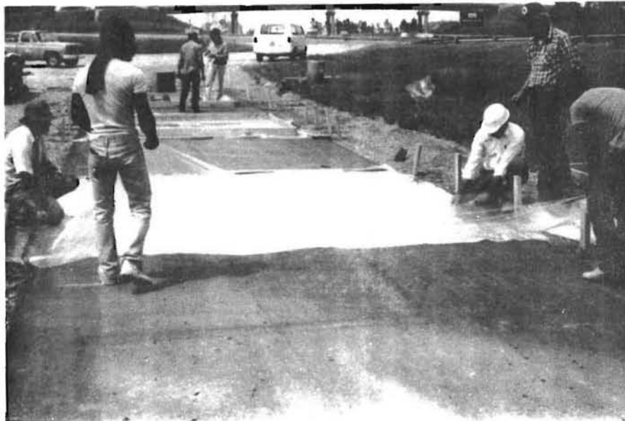
Fig 2.7. Placing of polyethylene sheeting on top of asphalt pad.
