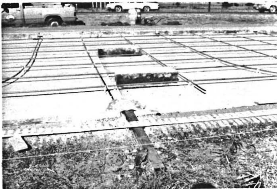
Fig 3.11. Blockouts for protecting embedded instrumentation; PVC conduit and steel channel section for protecting instrumentation leads.
