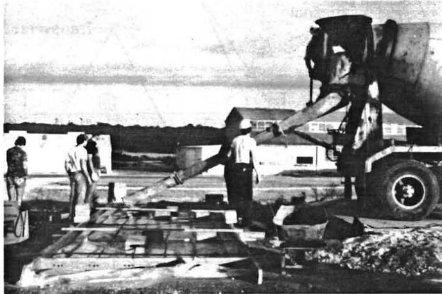
Fig 2.2. Concrete placement for the test slab.
