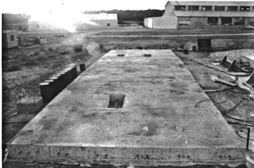
Fig 2.3. Test slab completed.
