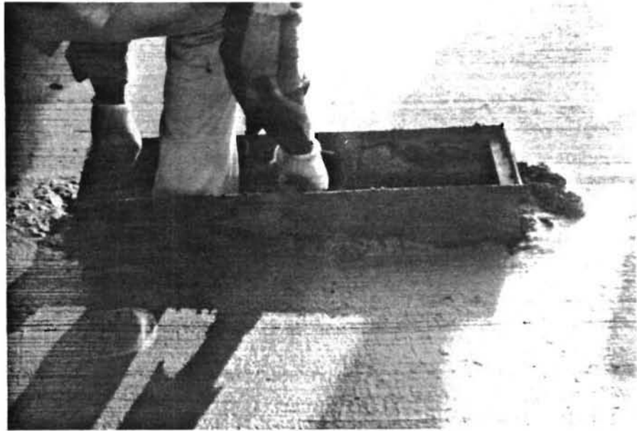
Fig 3.14. Removal of the instrumentation block-out after paving.
