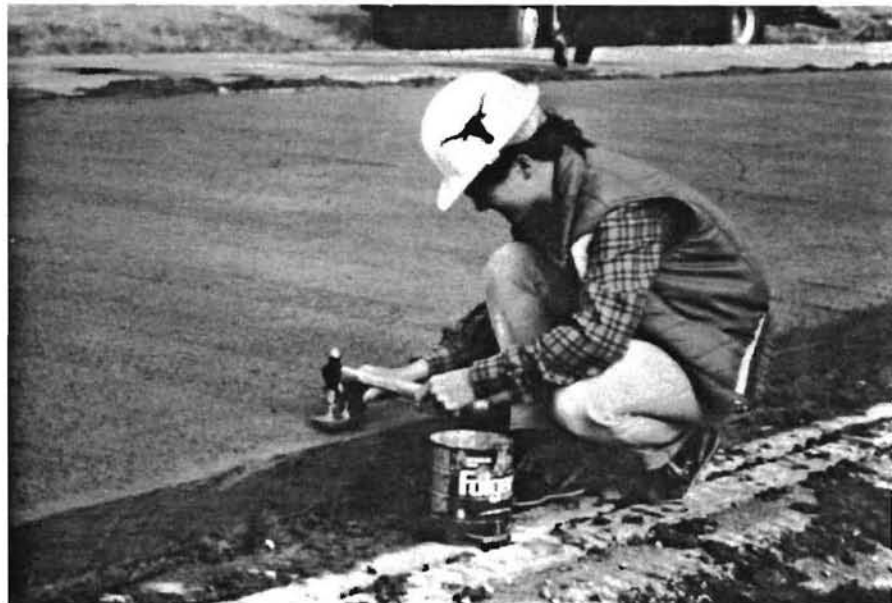
Fig 3.19. Attachment of steel angle for displacement transducer.
