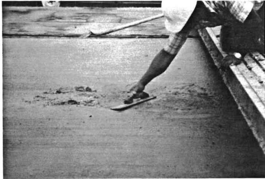
Fig 3.18. Finishing of concrete over embedded instrumentation.
