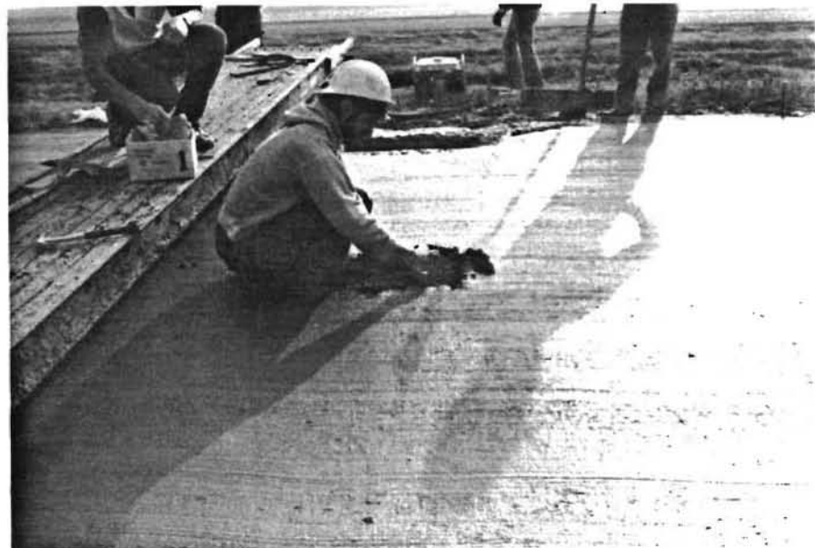
Fig 3.15. Final positioning of embedded gages.
