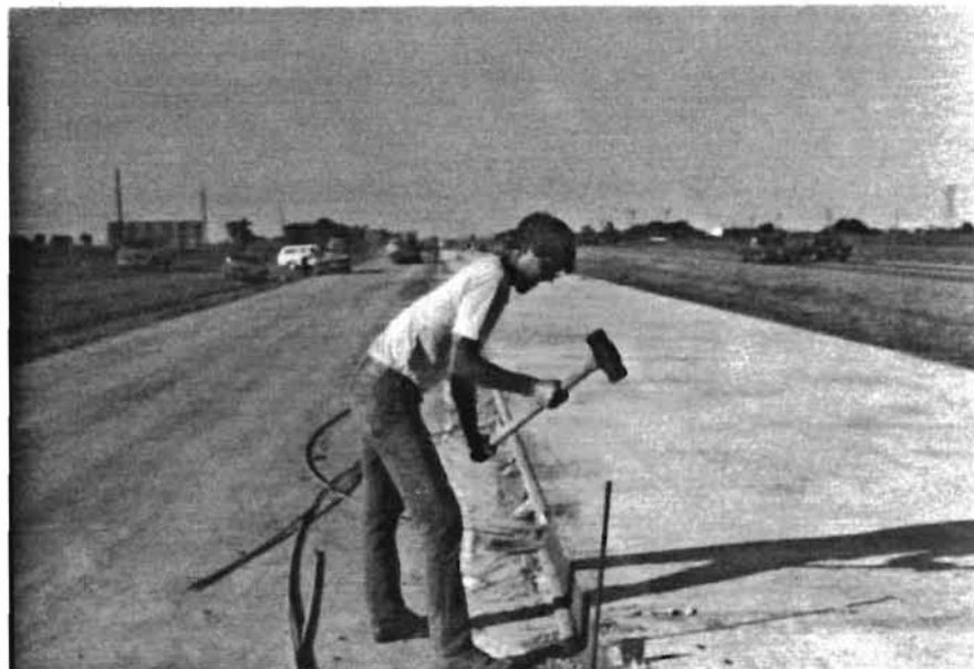
Fig 3.20. Installation of steel rod for mounting displacement transducer.
