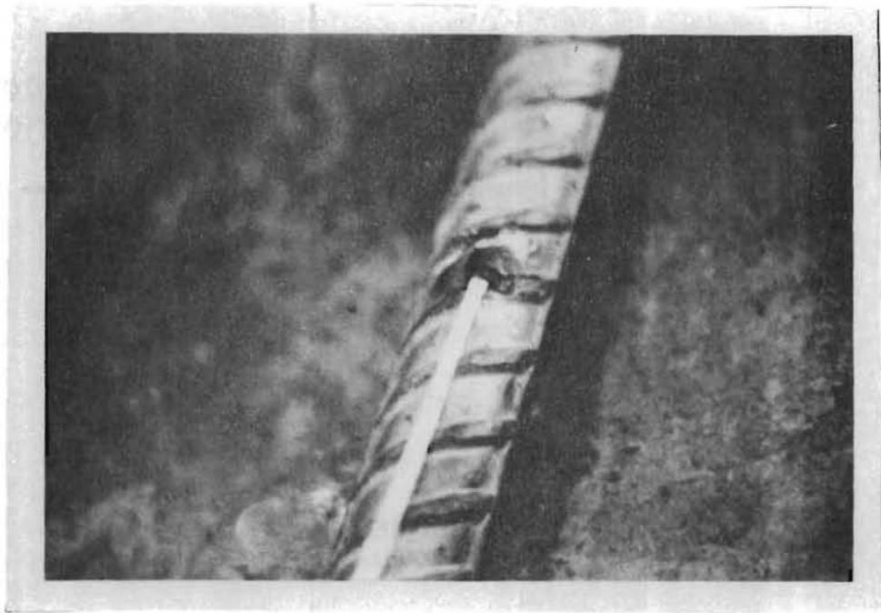
Fig. 3.4 Slip wire attached to pullout bar
