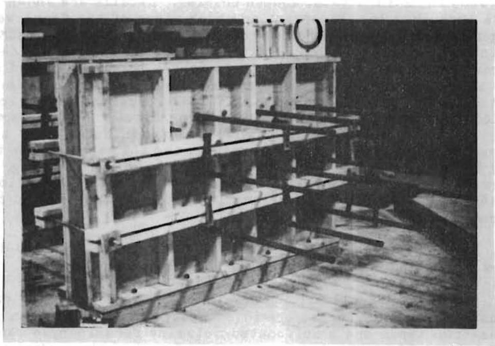
Fig. 3.7a Formwork ready for casting
