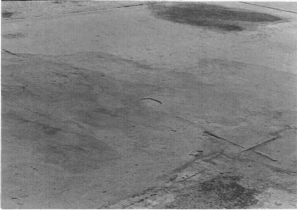
Figure 9. MMA repairs to area 2 are in good condition after six months.
