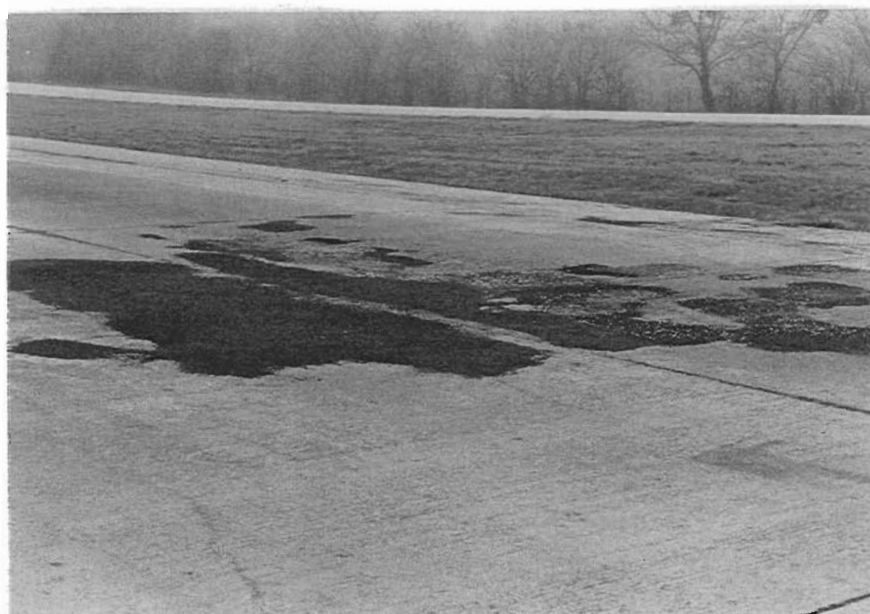
Figure 14. Overall condition of repair area 5 (slabs 41 and 42) is good.
