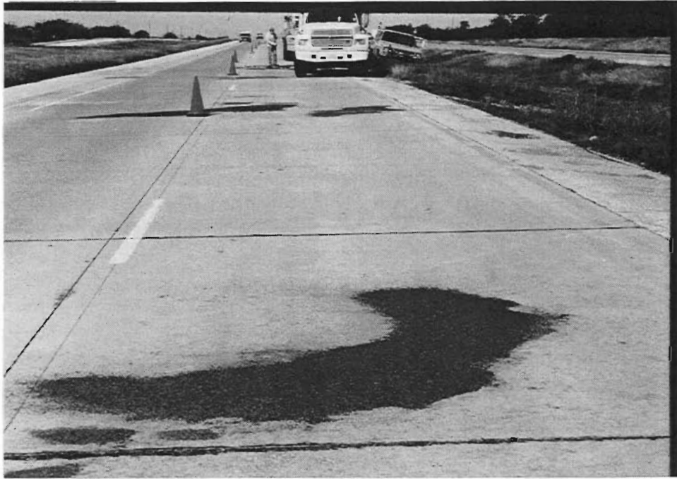
Figure 6. Area 4, consisting of slabs 22 and 23, shows no deterioration.
