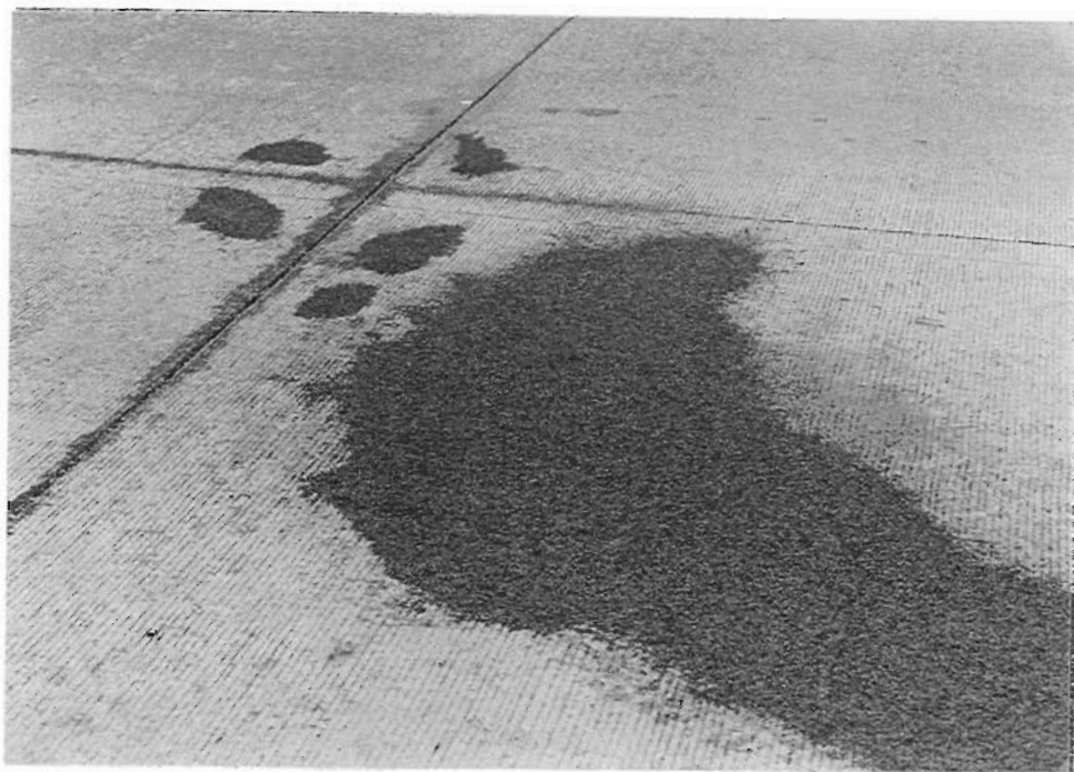
Figure 13. After one year, epoxy system in repair area 4 (slabs 22 and 23) shows no sign of deterioration.
