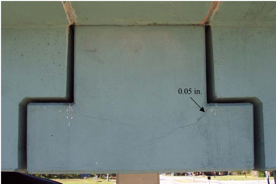
Fig. 4.4(b) Crack width at east end face of southeast inverted “T” bent cap at Laura Koppe Road
