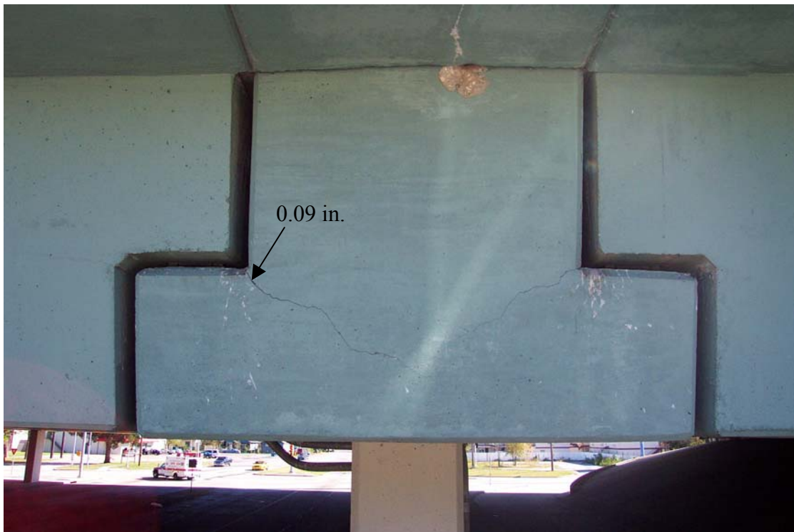
Fig. 4.4(a) Crack width at west end face of southwest inverted "T" bent cap at Laura Koppe Road
