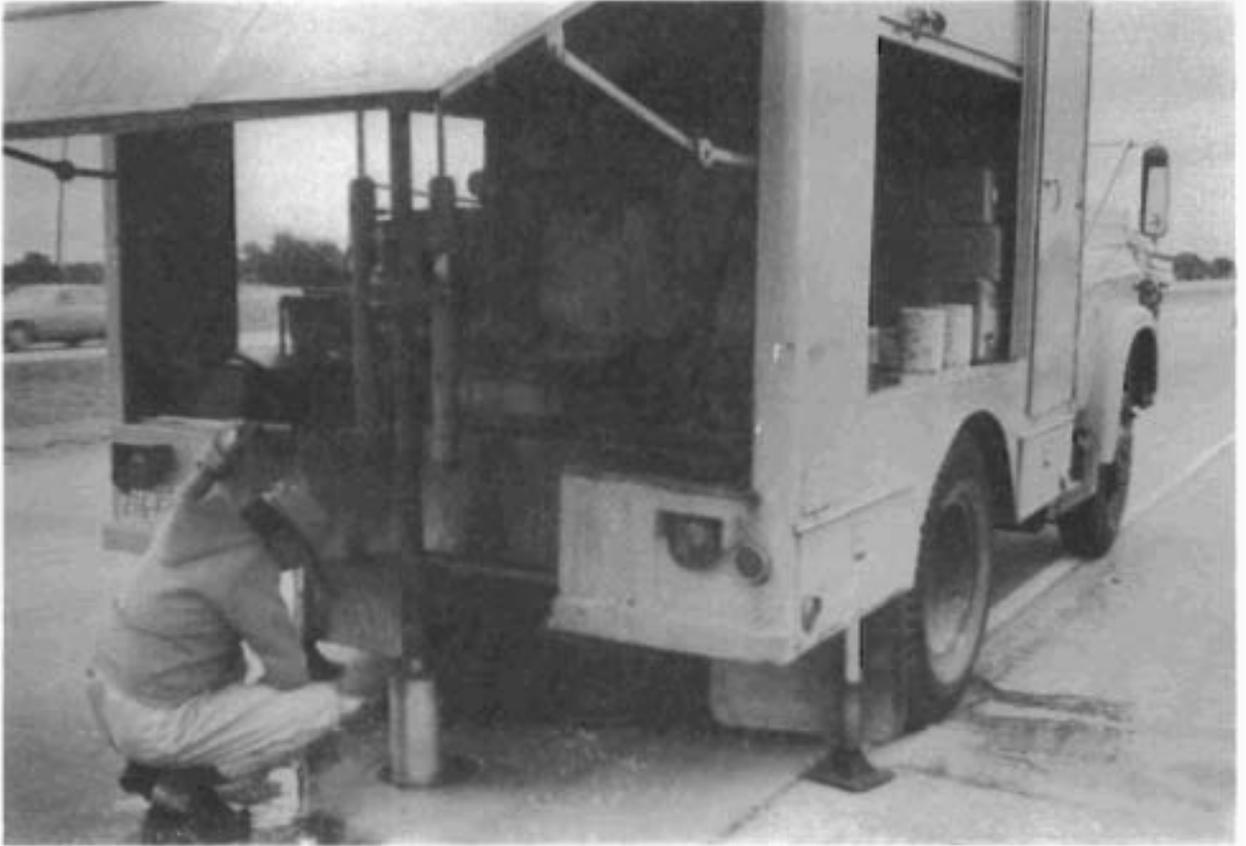
Fig 9. Coring operation.
