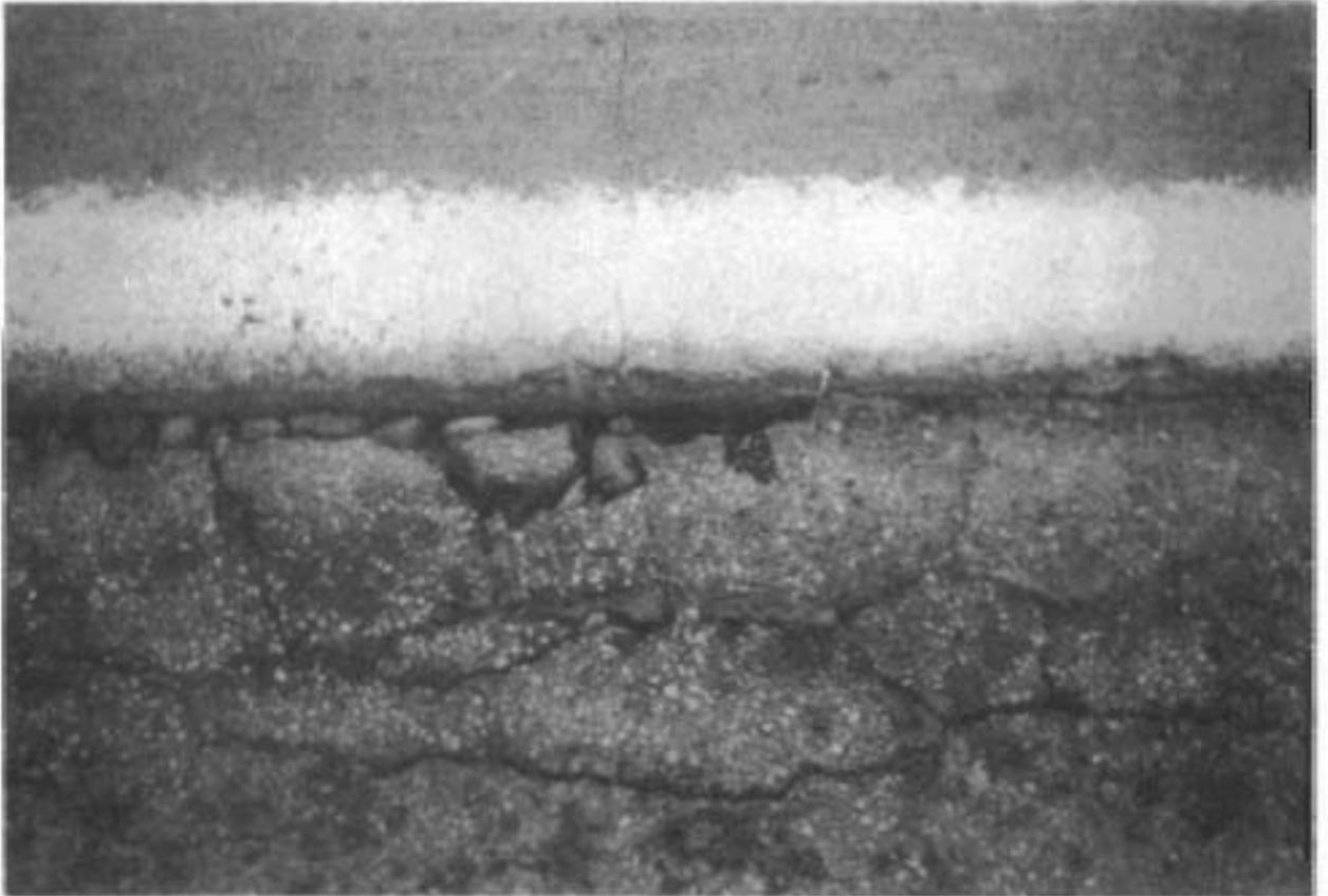
Fig 4. Severe edge pumping condition on CRCP.
