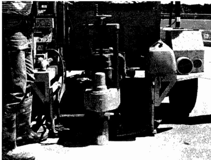
**Figure 4.10 Drilling of Concrete Core in Progress.**
