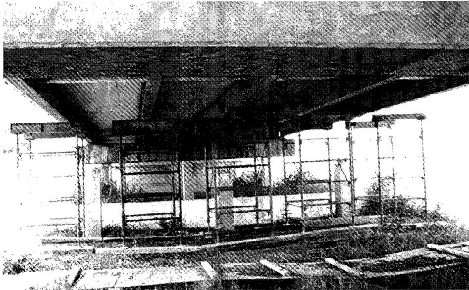
*Figure 5.2 Temporary Shoring in Place under Unit-N.*
