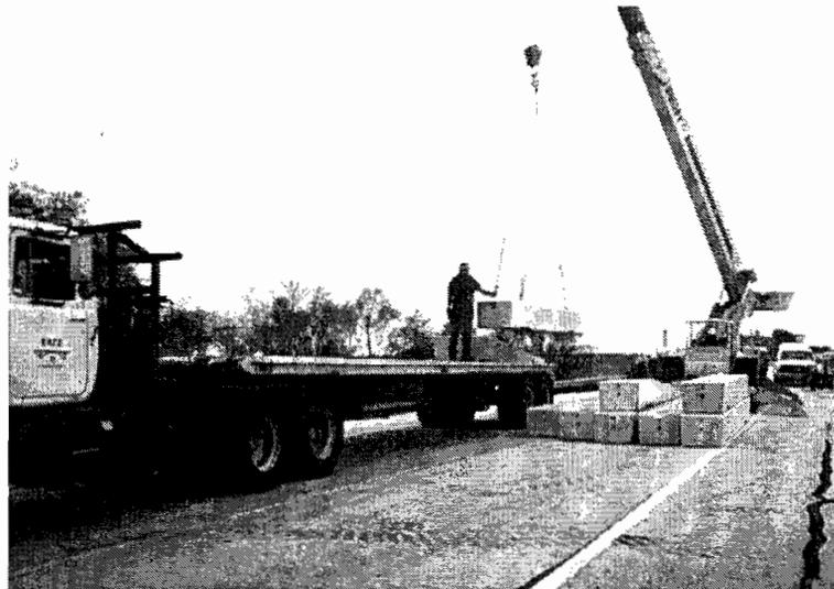
*Figure 5.8 Barrier Placement on Flatbed of Trailer.*
