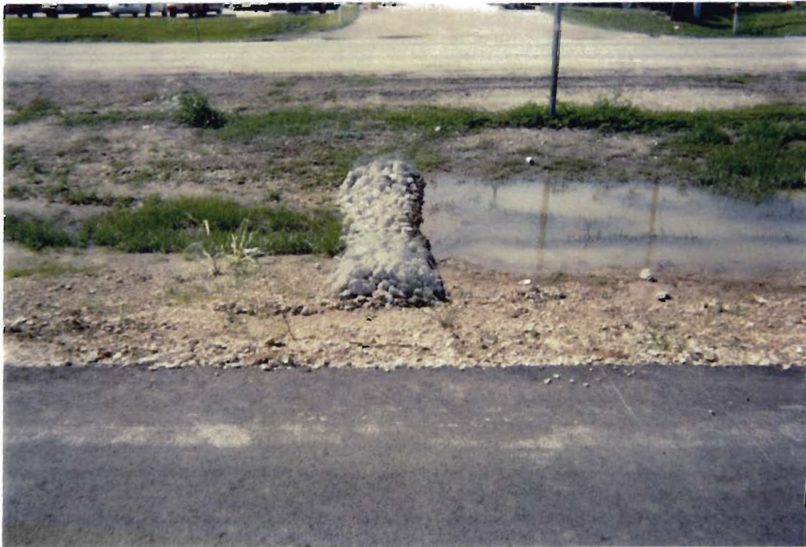
Figure 3: Rock Filter Dam TSC-3
