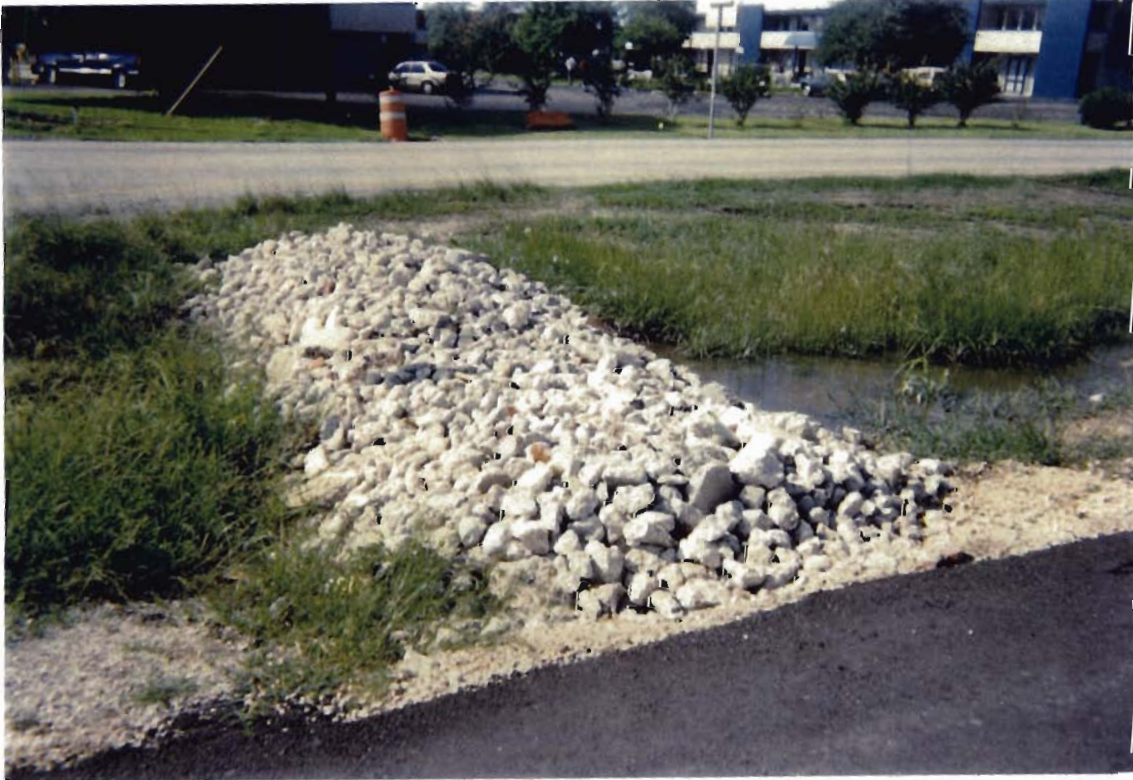
Figure 2: Rock Filter Dam TSC-1
