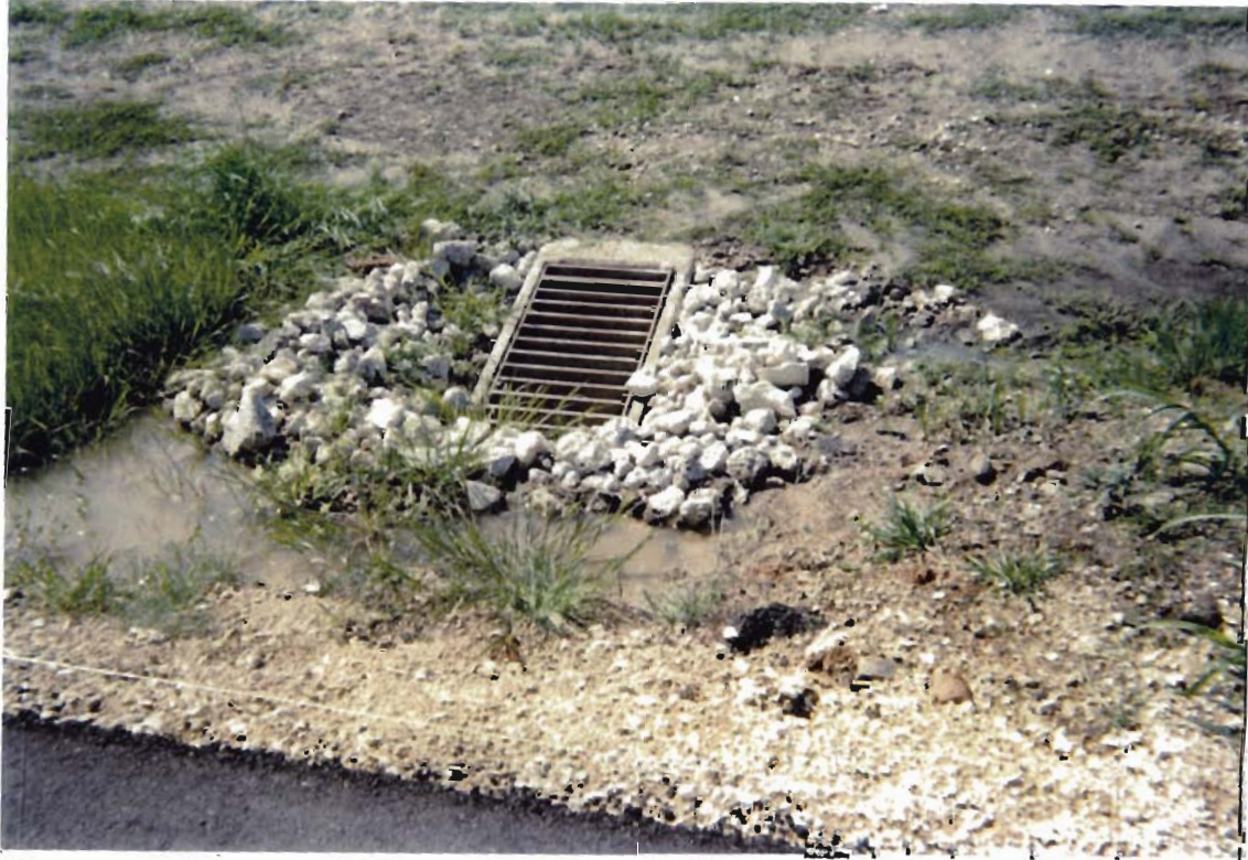
Figure 4: Rock Filter Dam TSC-4
