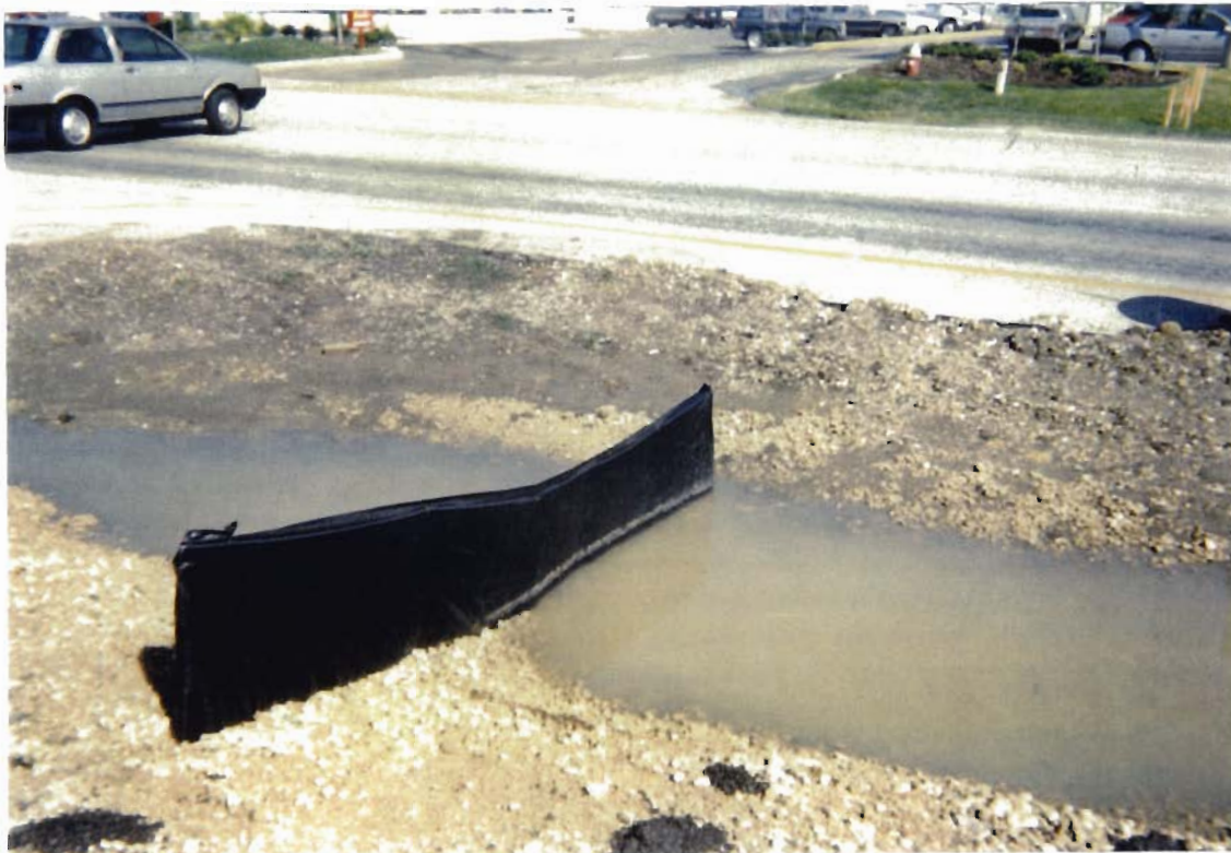
Figure 11: Sediment Control Fence with Runoff Flow around End of Fence Flowing onto Devegetated Area
