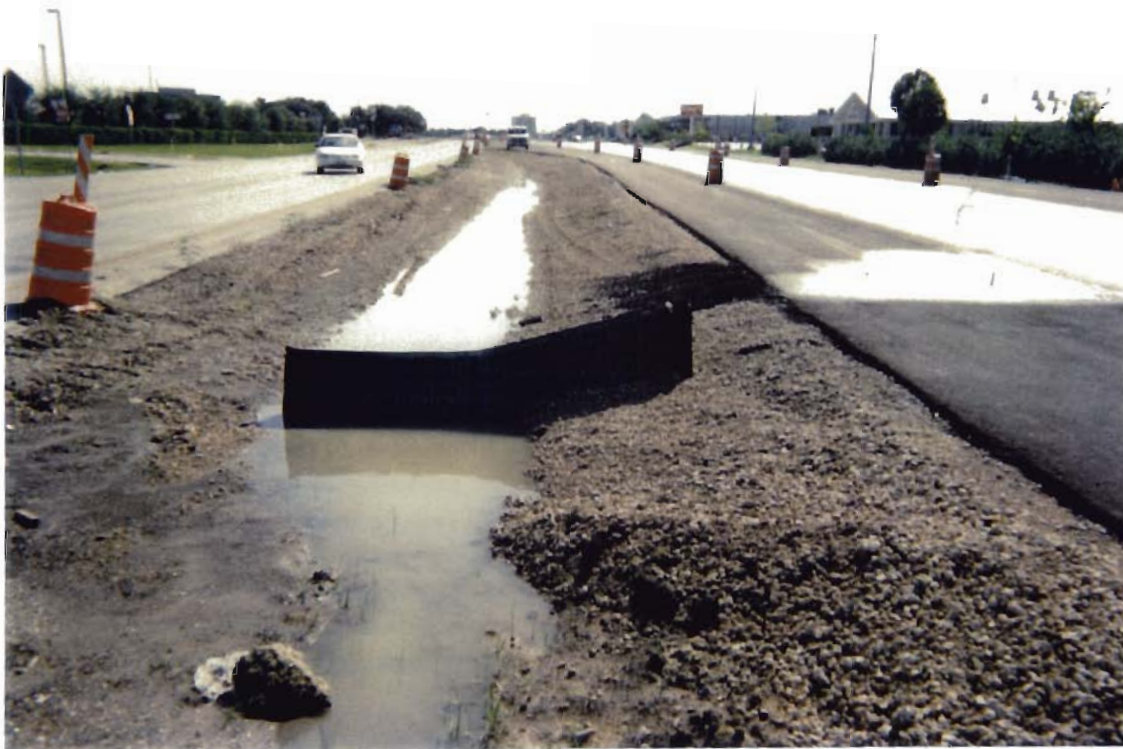
Figure 5: Sediment Control Fence TSC-2
