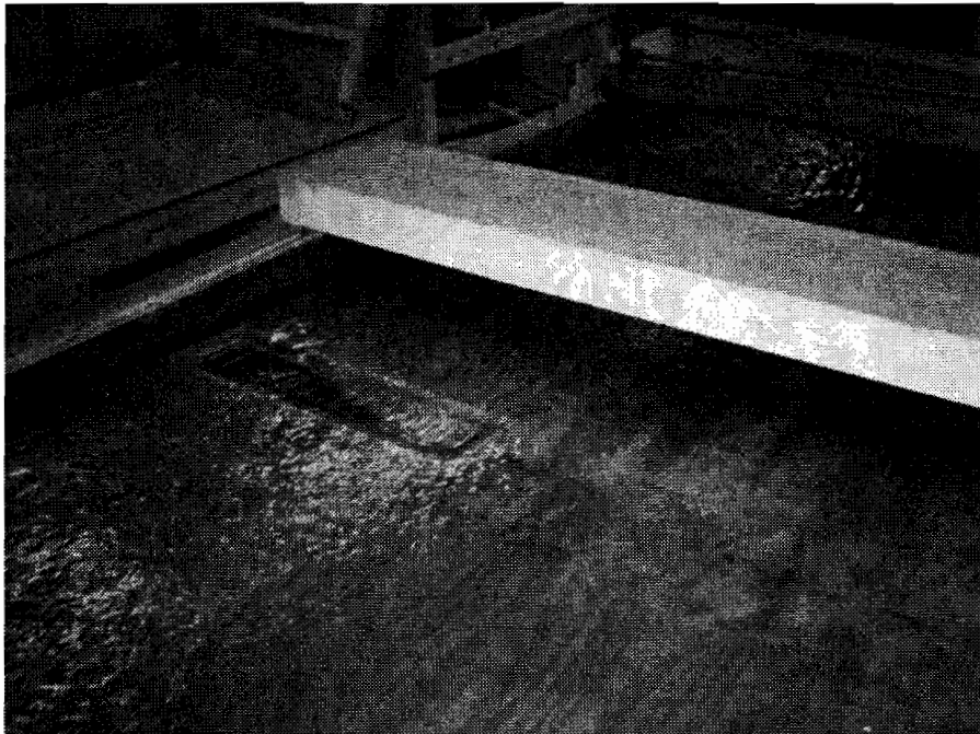
Figure C.3 Typical Test with Drain 2B, Looking Downstream
