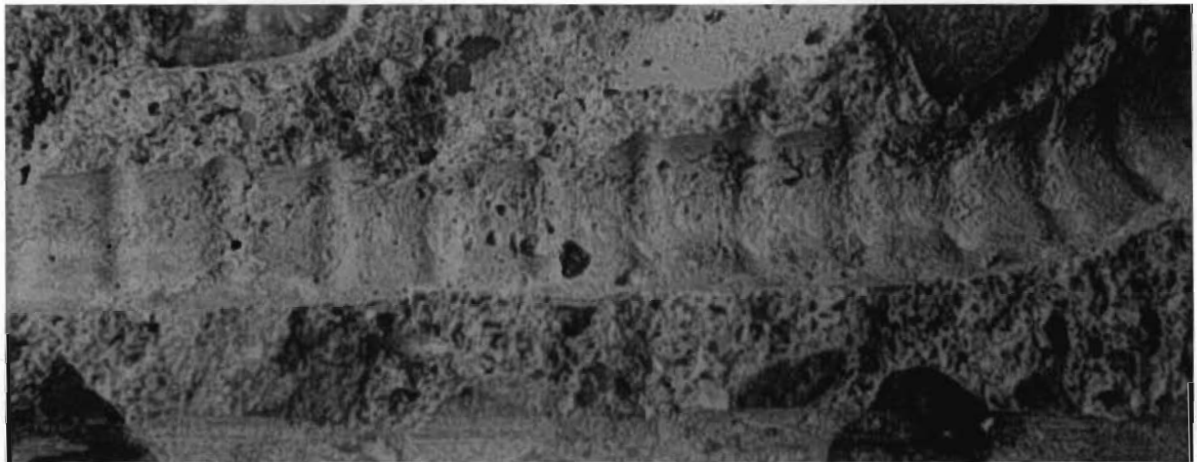
(b) Below the epoxy-coated bar.
