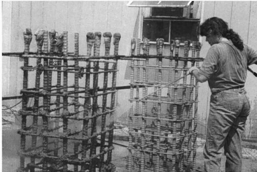
Figure 1.5 Washing column cages after vibration.
