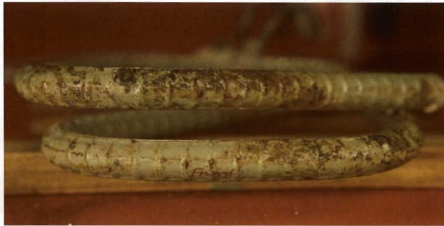
Figure 2.17 Rust staining of stirrup from beam B17.
