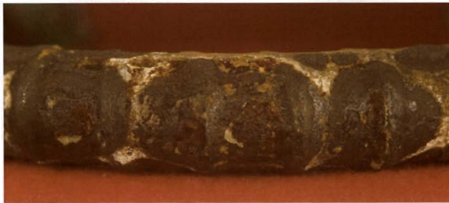
(b) Bar 2B.3 with unpatched damage at outside bend.
