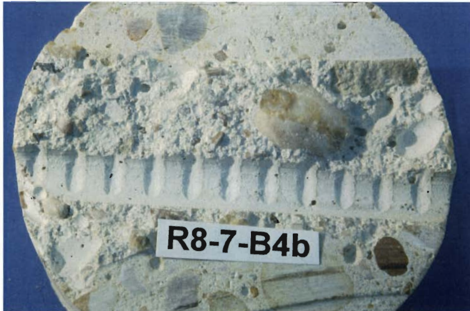
(a) Air voids close to point of vibrator insertion.
