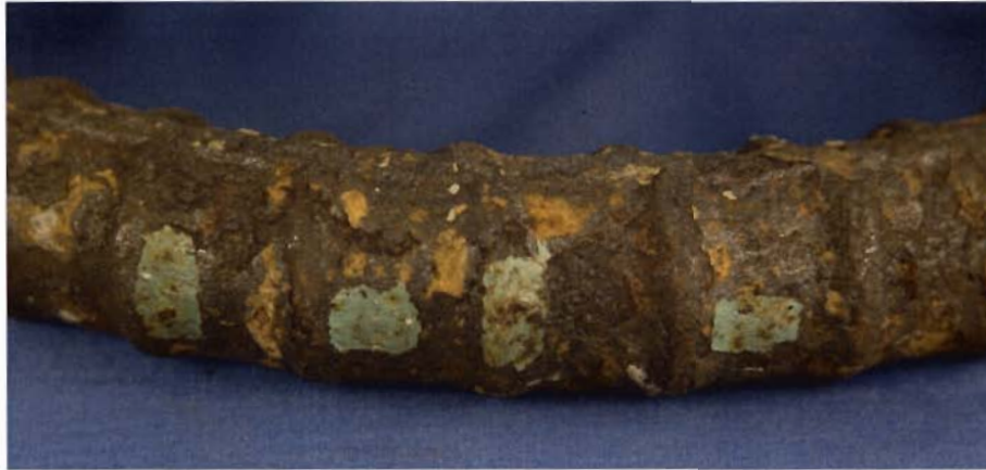
(a) Patched bar 3B.2, outside bend.
