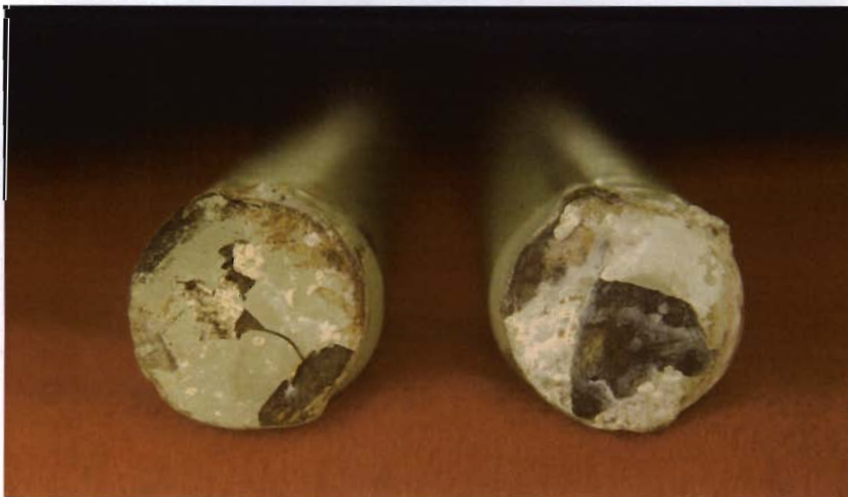
Figure 3.2 Patch at bar ends of splice bars broke during autopsy, showing a dark corroded surface underneath after 4.3 years of exposure (beam study).
