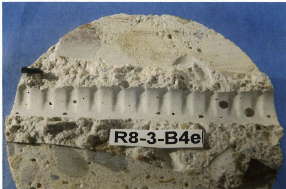
(b) Air voids farther away from point of vibrator insertion.
