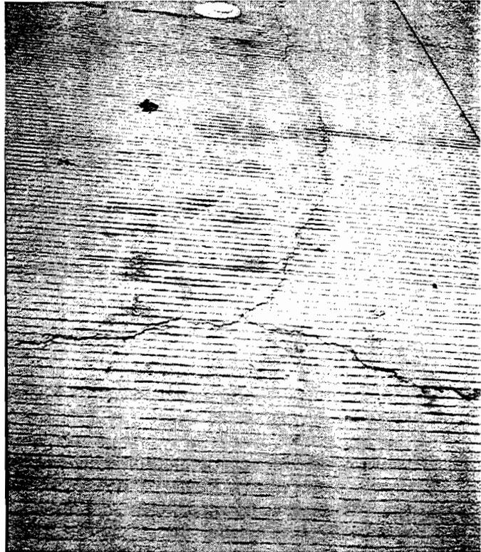
*Figure 4.9 Typical longitudinal crack occurring with summer placements (SH 6 summer)*
