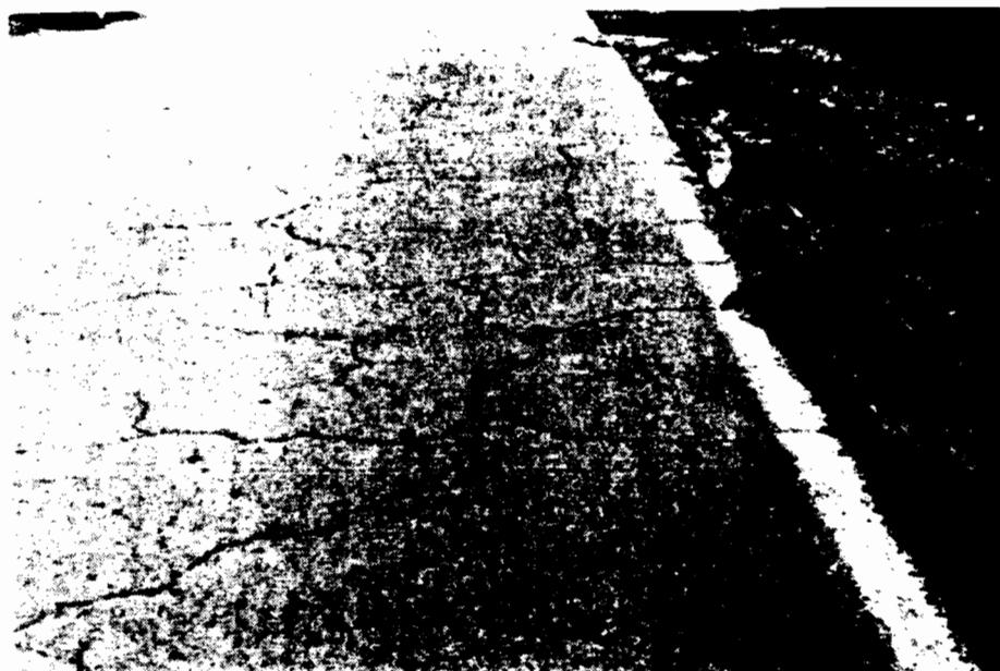
Figure 1.5 Block cracking
