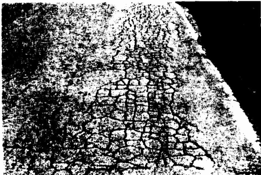
Figure 1.4 Alligator cracking
