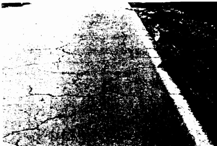
Figure 1.5 Block cracking
