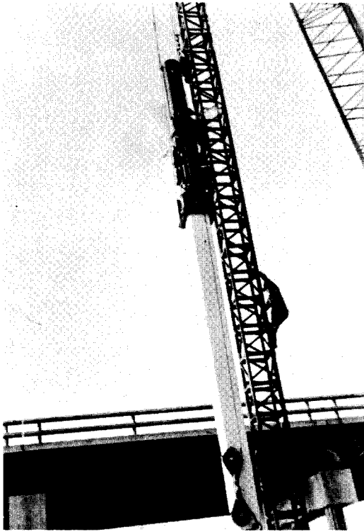
Figure 6. Delmag D-22 diesel hammer driving prestressed concrete pile.
