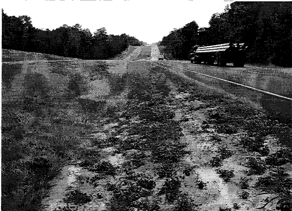
Fig 2.3. General site description of flexible pavement test section.
