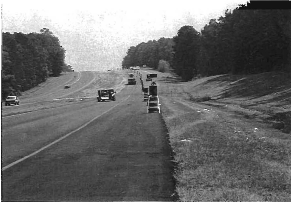
Fig 4.9 Plastic barrels as channeling devices at Work Zone 2.
