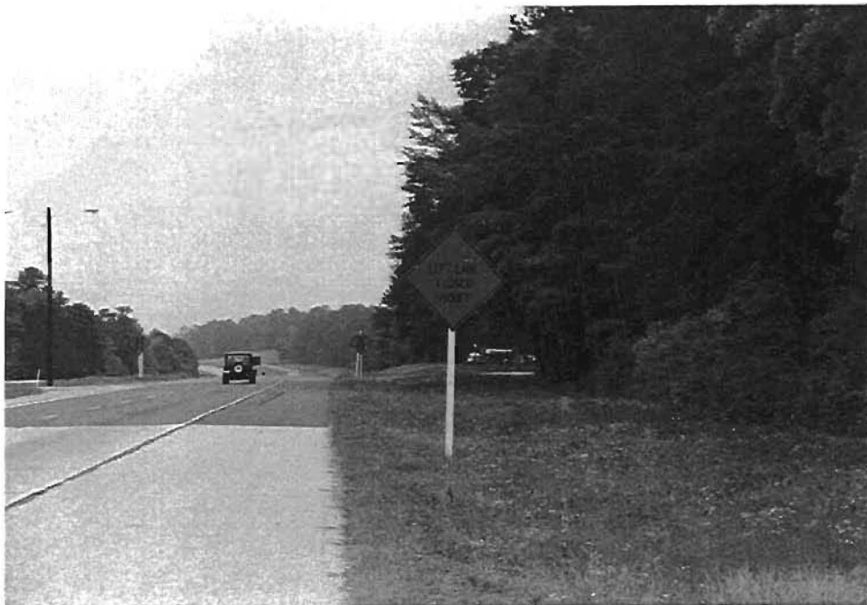
Fig 4.5. Traffic signs for Work Zone 1 on northbound lane (4/9/92).
