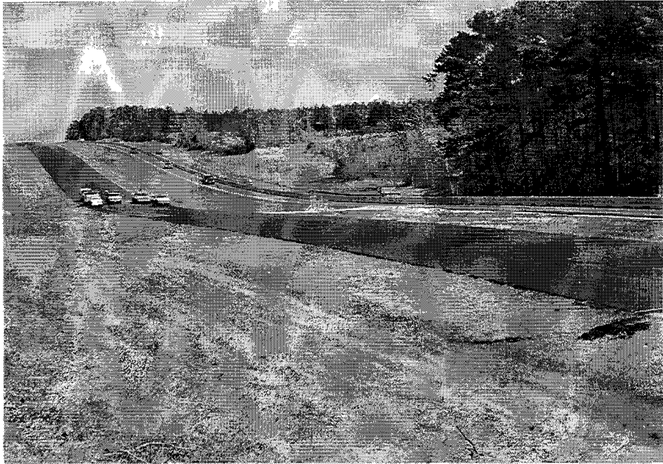
Fig 2.2. General site description of rigid pavement test section.
