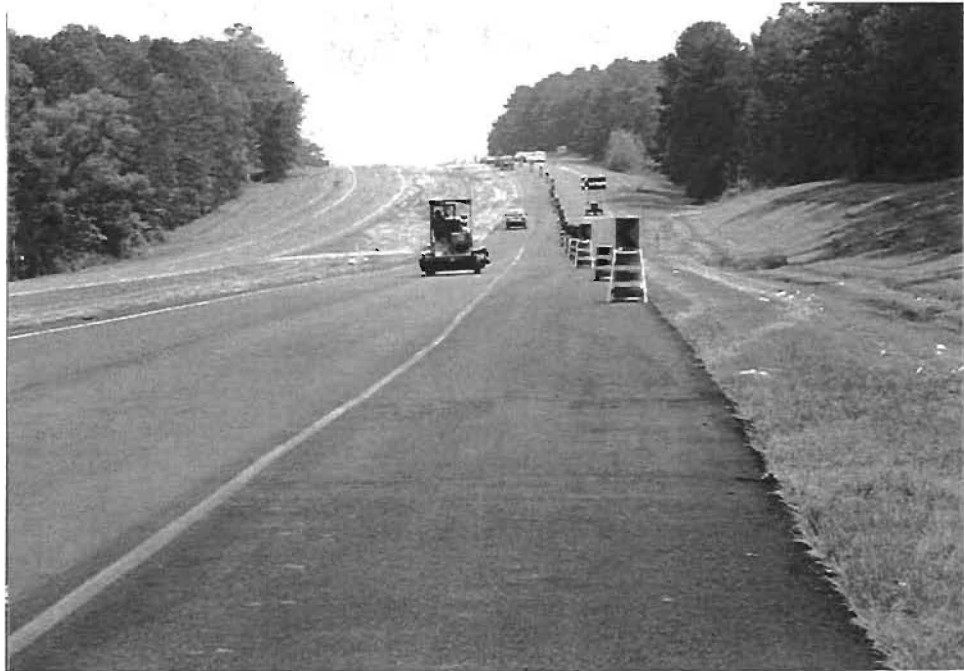
Fig 4.10 Arrow panels at Work Zone 2 on the southbound lane (6/23/92).
