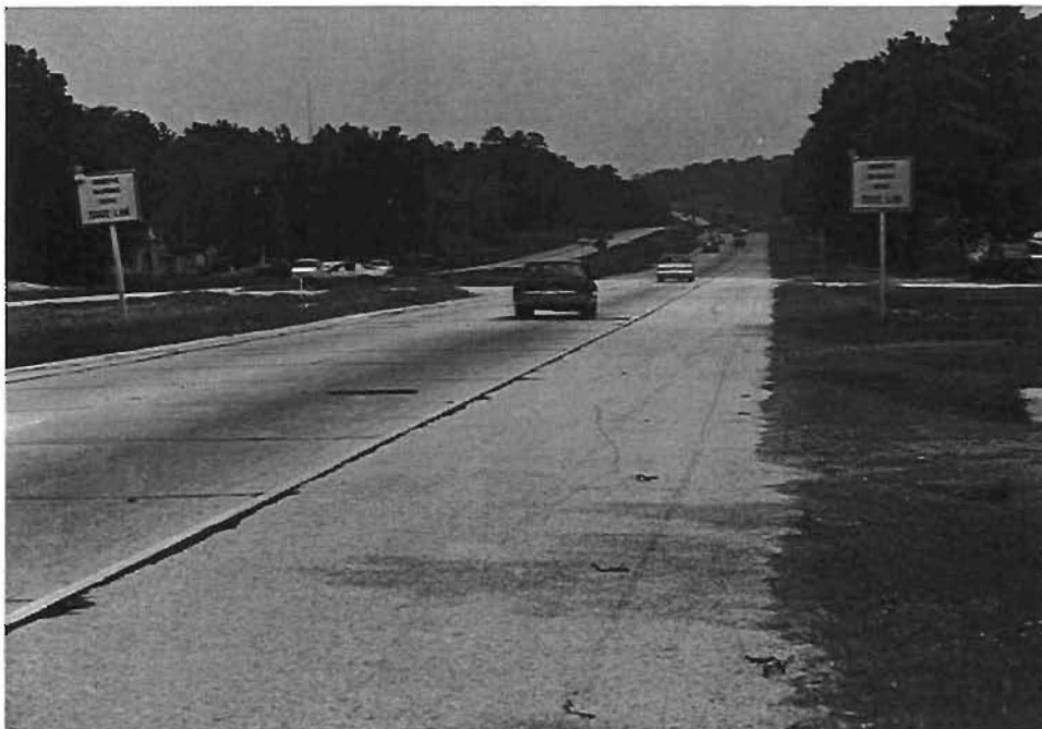
Fig 4.3. Traffic signs for Work Zone 1 on the northbound lane (4/9/92).
