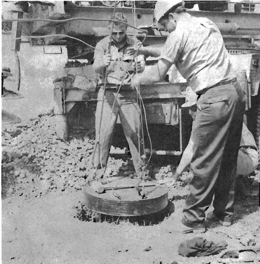
Fig. 4.3. Placing of Bottomhole Cell
