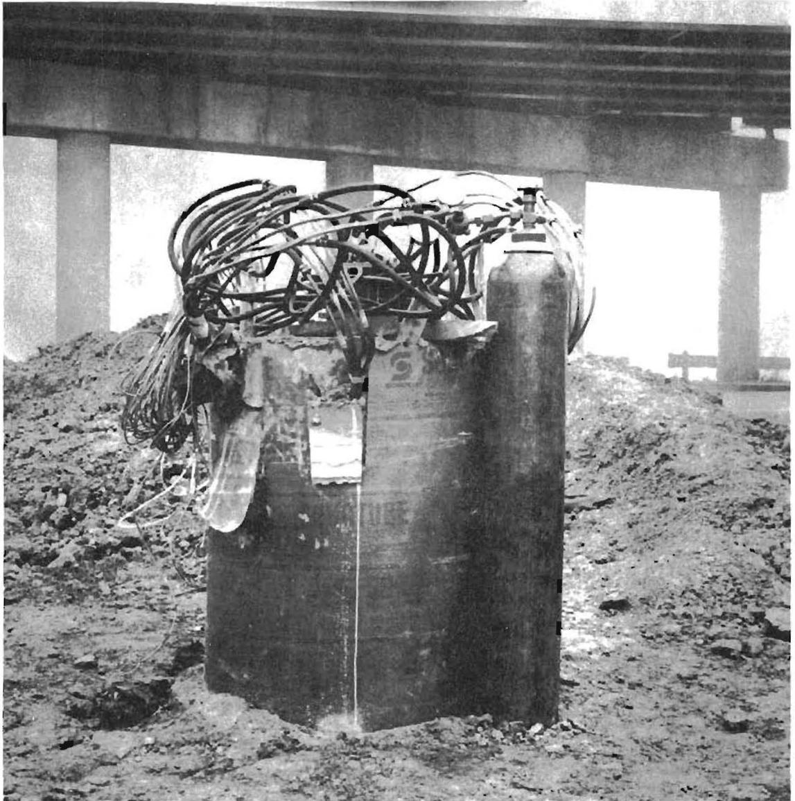
Fig. 4.25. Shaft Head and Mustran Manifold System,
