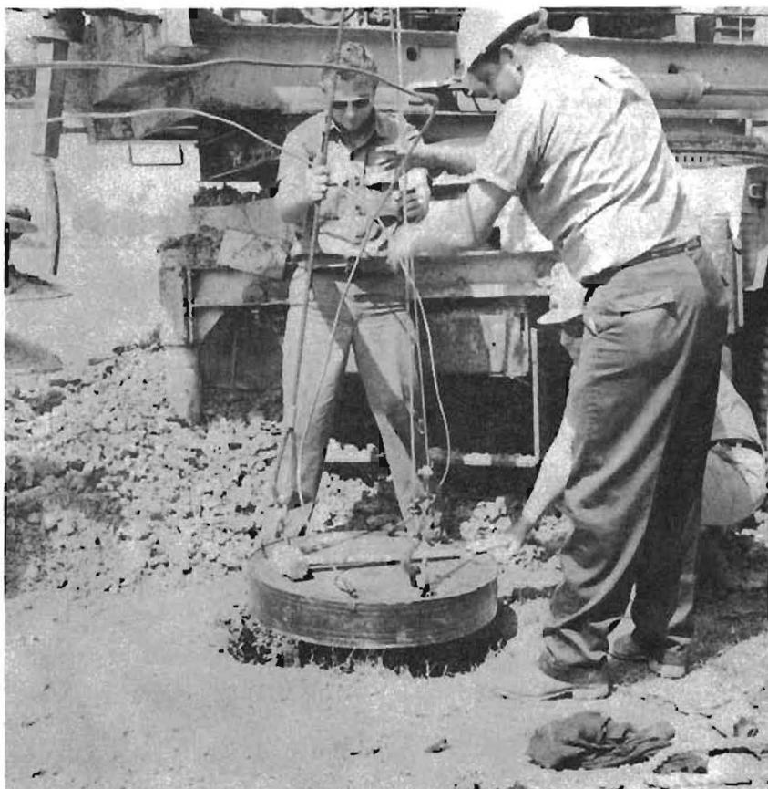
Fig. 4.3. Placing of Bottomhole Cell
