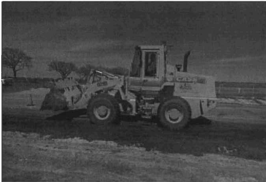
Figure 5.4 Distributing Composts on the Tilled Subgrade
