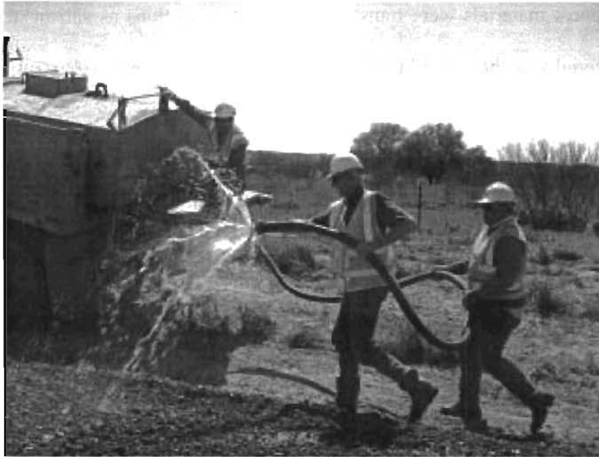
Figure 5.5 Application of Water over the CMT Loose Mixture
