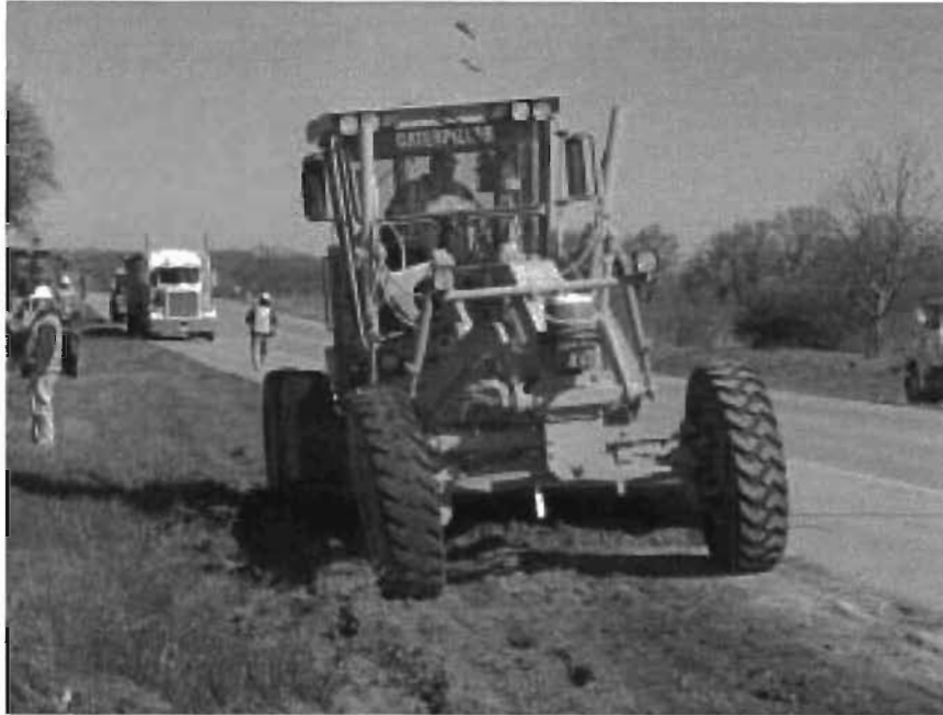
Figure 5.2 Maintainer to Blade the Subgrade Shoulder
