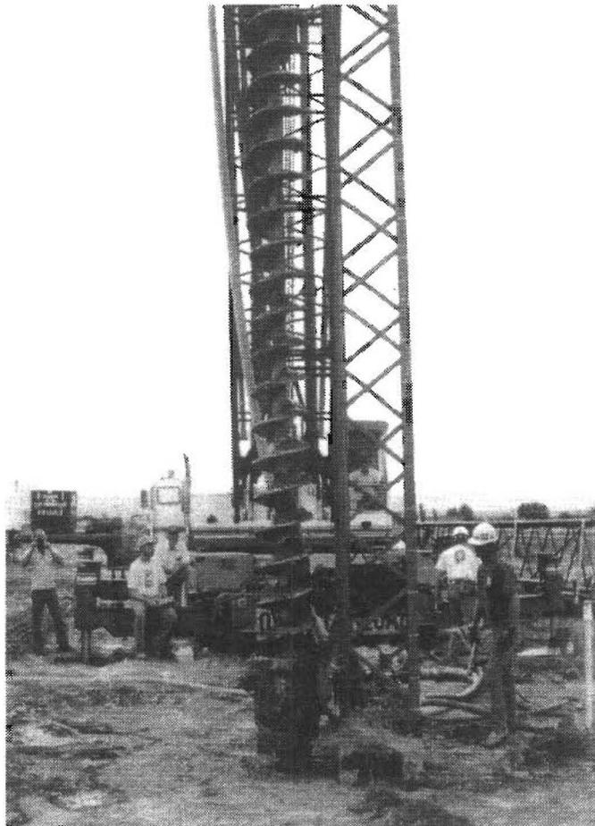
**Fig. 6.2. Positioning continuous flight auger.**
