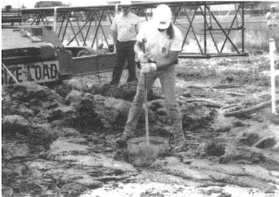
**Fig. 6.8. Removing clods of loose soil from grout column.**
