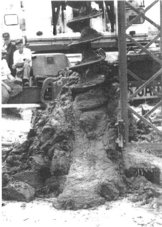
**Fig. 6.7. Auger immersed in grout after completion of grouting operation.**
