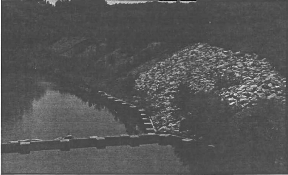
Figure 15. Grade control structure on the downstream side of the bridge crossing Bear Creek on the Northbound Spur 97 in Tarrant County.
