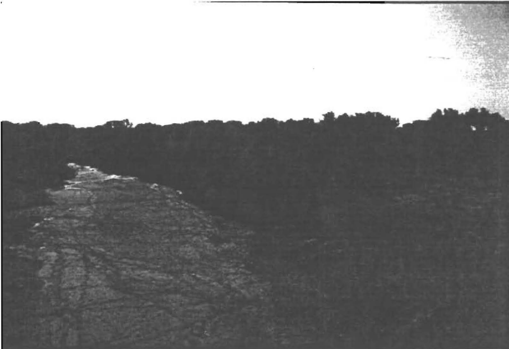
Figure 24. Channel of the Pease River immediately upstream from the crossing on State Highway 6 in Hardeman County showing accelerated bank erosion by livestock entering the channel adjacent to the northern abutment.
