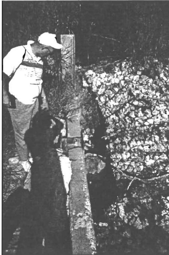
Figure 14. Intensified erosion on the downstream side of the drop structure required installation of wire basket gabions for erosion control, which are now failing because of foundation problems.
