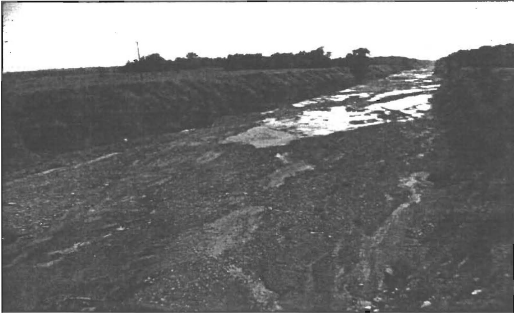
Figure 21. Photograph with a view east to show a view of the channel downstream from the bridge. Natural channel alluvium has been scoured away by erosion. The banks are subject to slope failure and to erosion. The channel bottom is bedrock with a few scattered gravel drifts over the surface.
