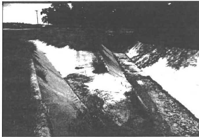
Figure 22. Modifications to an unnamed tributary of the Navosota River near SH 6 in Brazos County. The drainage way on the left drains highway runoff toward the observer and makes a left hand turn into the drainage channel to the right which transports runoff from the watershed east of the highway. This channel flows away from the observer to a sharp curve where the concrete channel ends and an earthen channel starts at the top of the photograph.
