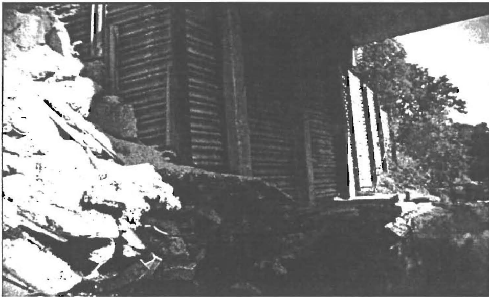
Figure 10. Concrete rubble dumped on the upstream upside of the abutment was covered in-place with poured concrete in an attempt to slow erosional retreat of the bank. Such “unconventional” measures pose an aesthetic and perhaps an environmental concern.
