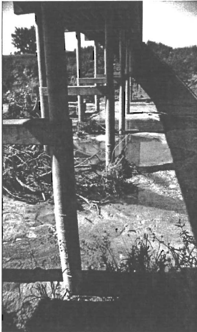
Figure 20. Photograph of view north to show the channel cross section at the bridge. The level of the channel at the time the piers were poured can be seen on by the markings on the two closest piers. Erosion of the channel bed is endangering all the bridge support structures and both abutments.
