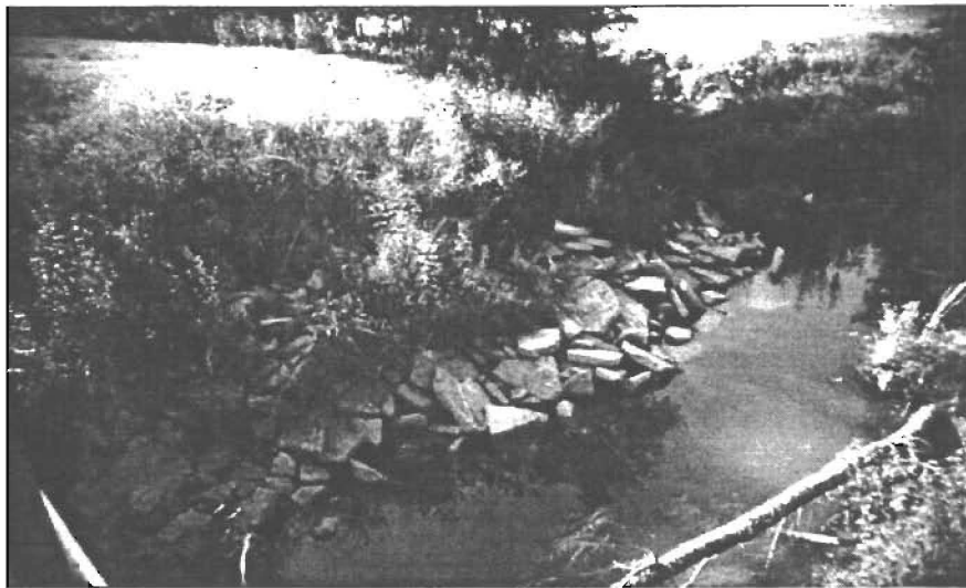
Figure 7. FM 1550 bridge crossing Brushy Creek in Fannin County (above) with concrete rubble dumped to mitigate impingement of flows on west channel bank and abutment of bridge.
