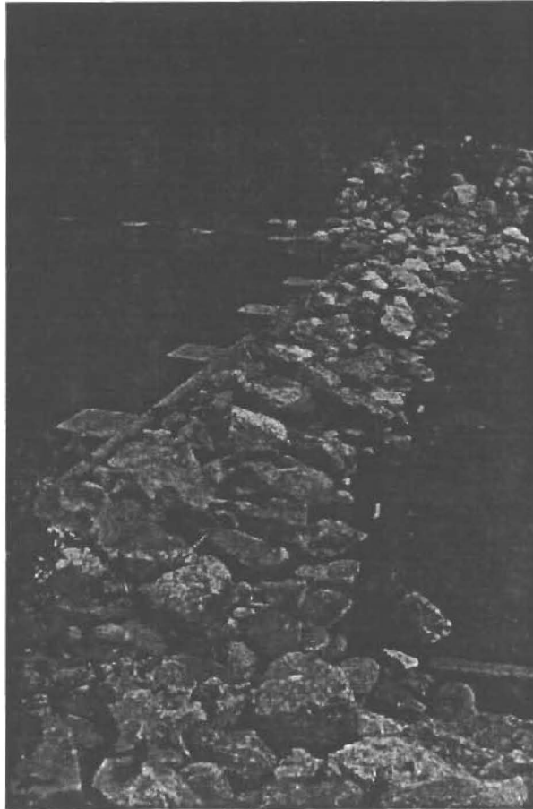
Figure 16. Downstream side of the grade control structure.
