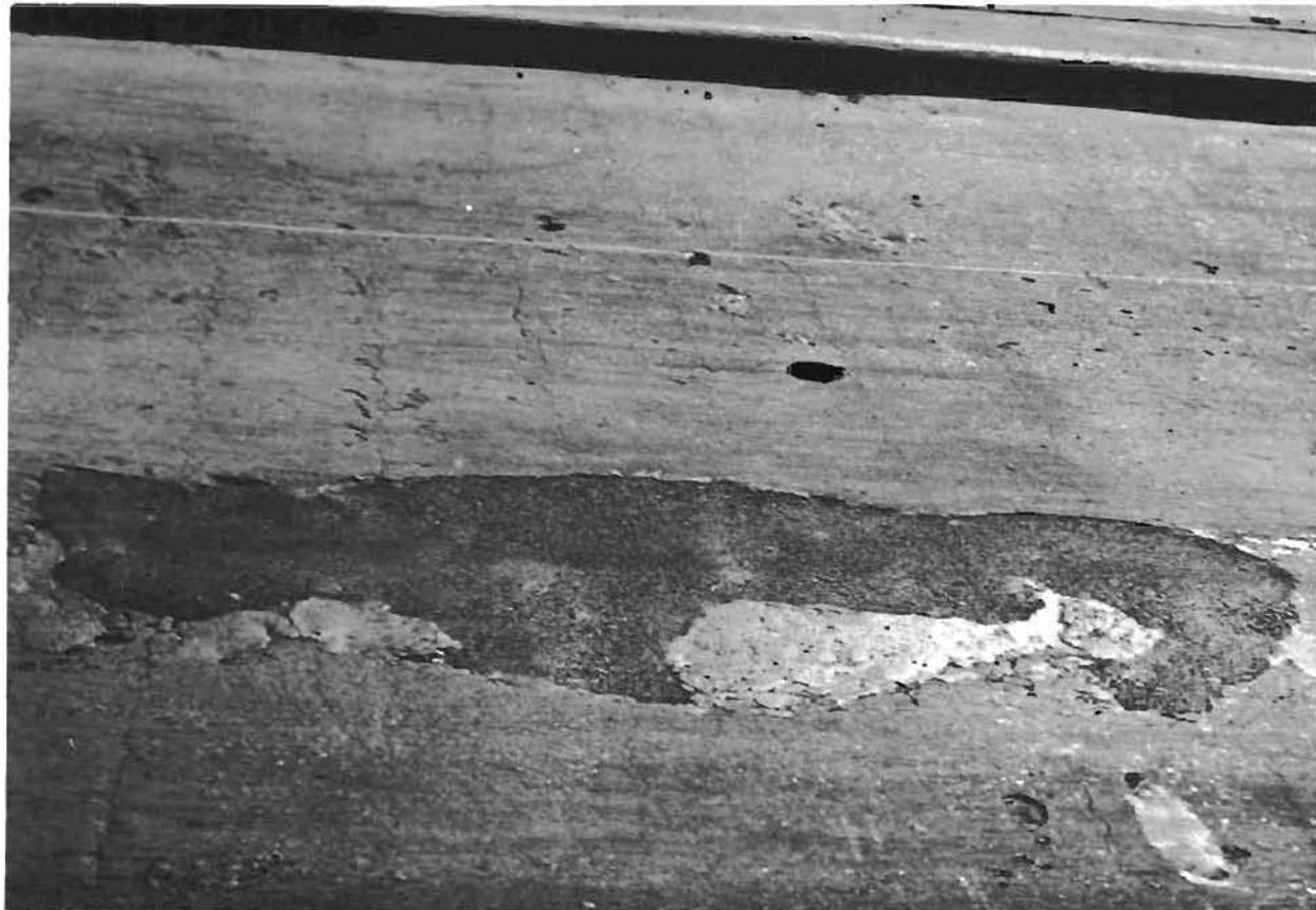
FIGURE 3 CRACKING AND SPALLING OF SLAB
