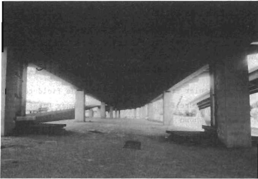
Fig. 2.1 Underview of a twin girder steel bridge
