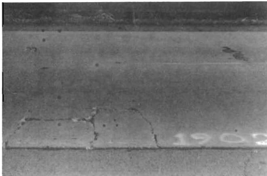
Fig. 7.21 Marshall Repair No. 2 Before Cracks Widened
