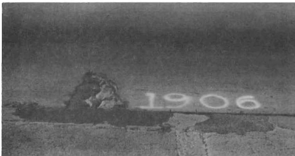
Fig. 7.23 Marshall Repair No. 4 Prior to Removal of Concrete
