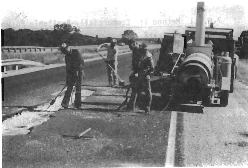
Fig. 7.32 Drying of Repair No. 1
