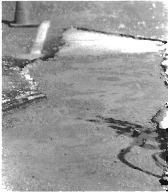
Fig. 7.42 Completed Repair using User-Formulated PC
