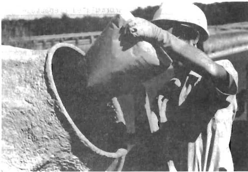
Fig. 7.33 Transfer of Powder Component into Concrete Mixer
