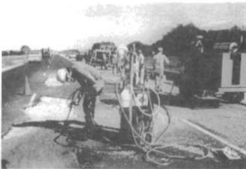
Fig. 7.40 Injecting Monomer into Premixed Aggregate using In-Line Mixing System
