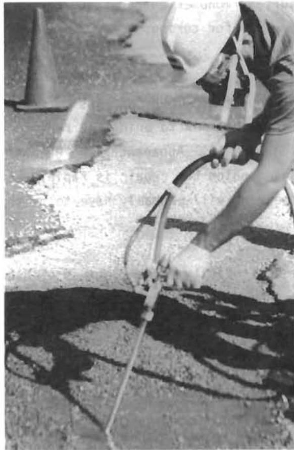
Fig. 7.41 Close-up View of Monomer Injection into Premixed Aggregate
