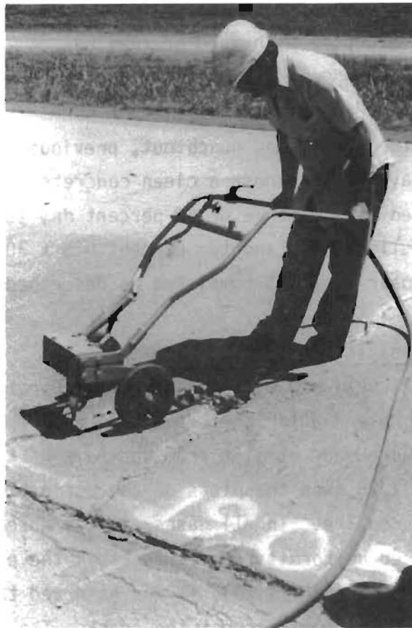
Fig. 7.24 Cracks in Repair No. 3 Opened with Crack Chaser
