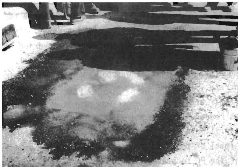
Fig. 7.30 Completed Repair at Comanche
