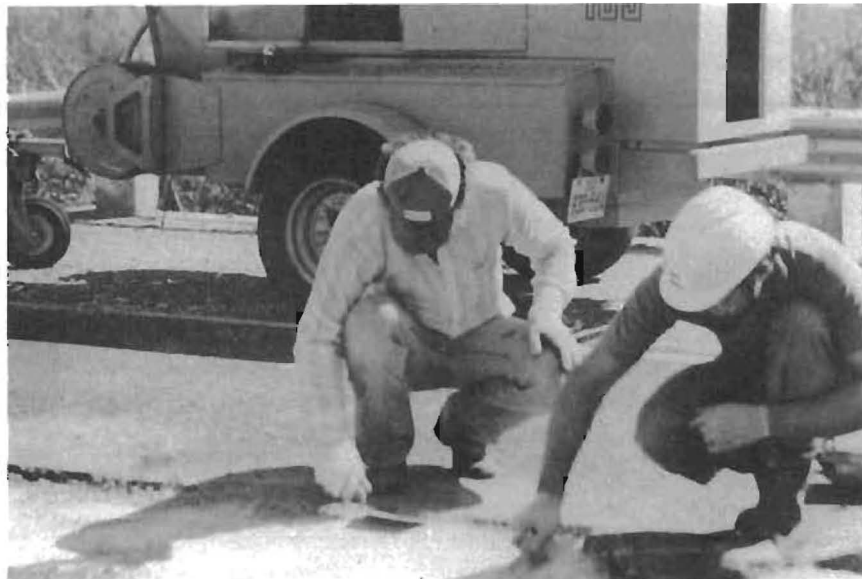
Fig. 7.36 Finishing the Surface of User-Formulated Prepackaged PC
