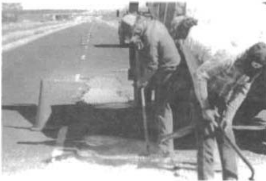
Fig. 7.39 Placement of Premixed Aggregate into Repair Hole No. 2
