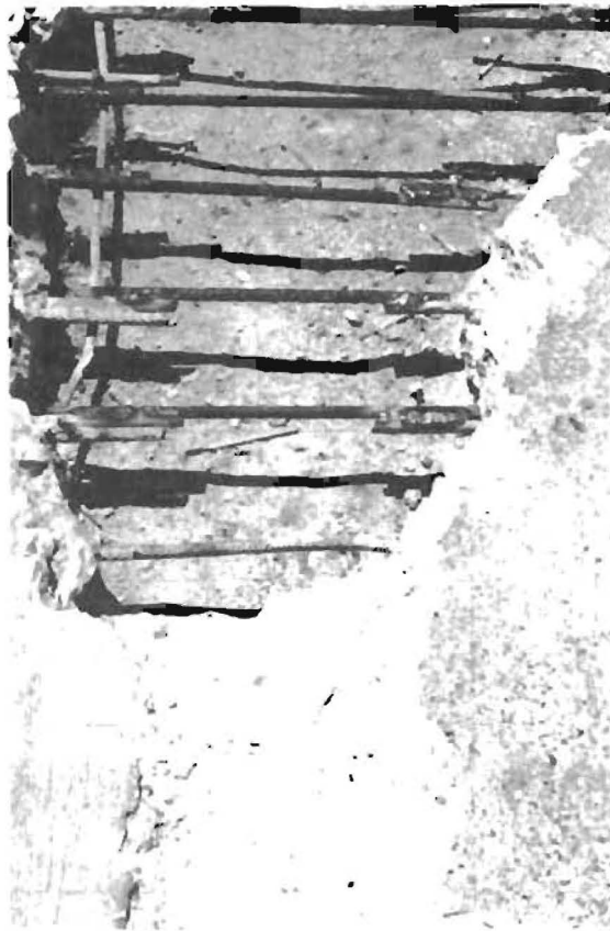
Fig. 7.20 Marshall Repair No. 1 After Removal of Asphalt
