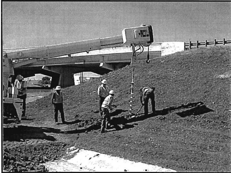
**Figure 11. Drilling Boreholes at Motley Drive Site**
