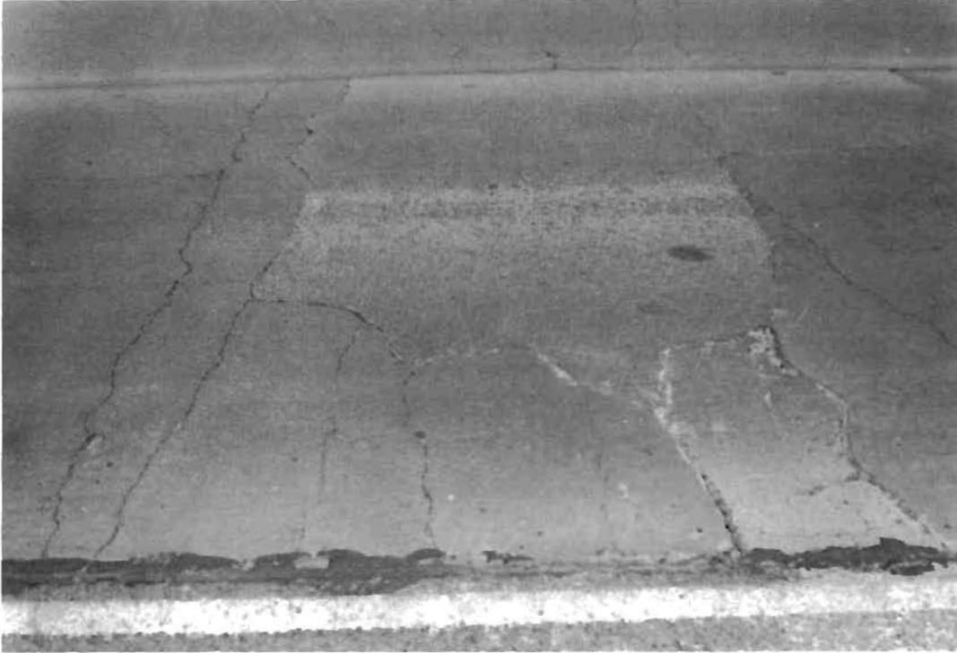
Fig 1.1. Portland cement concrete patch with further deterioration adjacent to patch.
