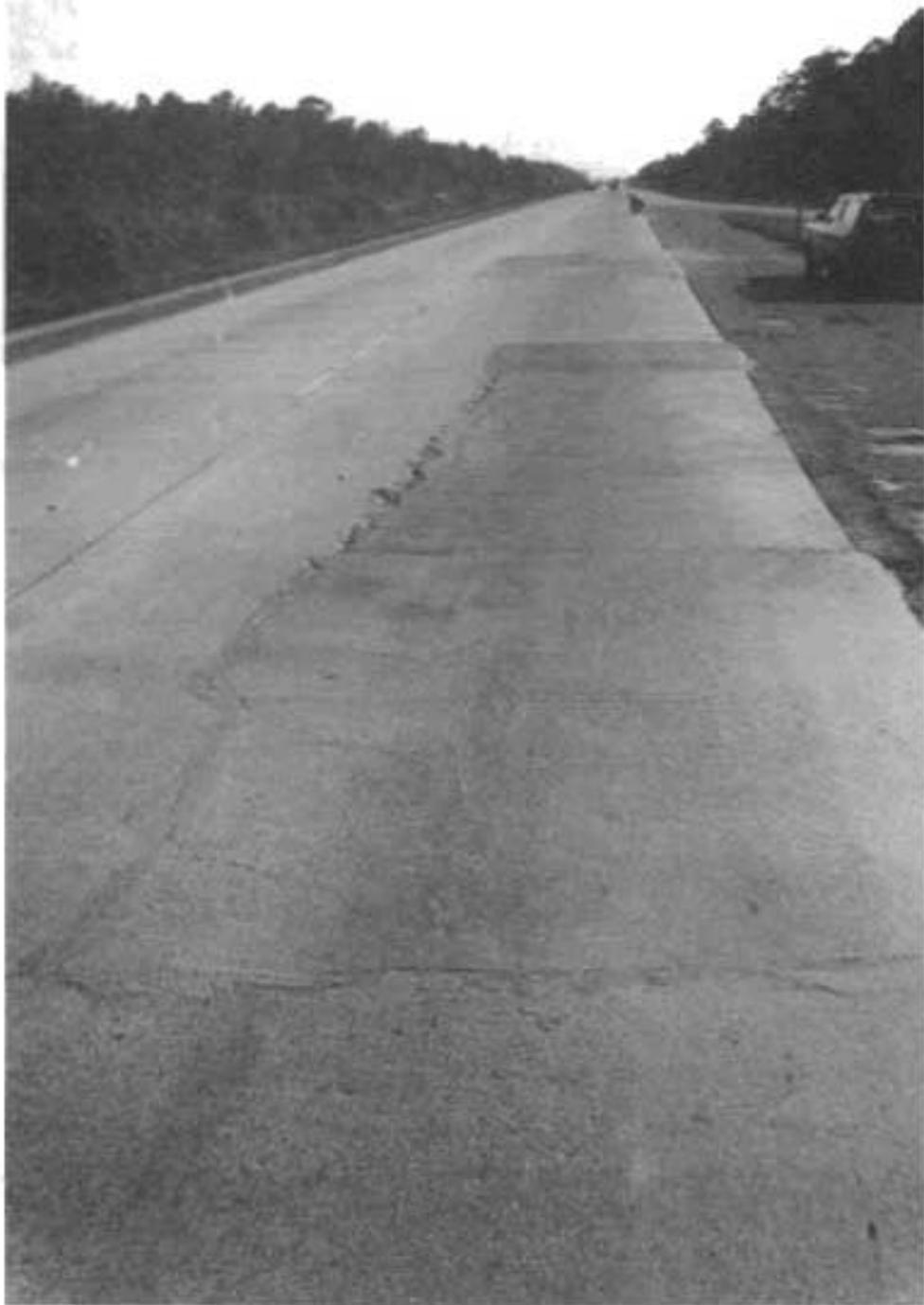
Fig 2.4. Portland cement concrete patches placed side by side.
