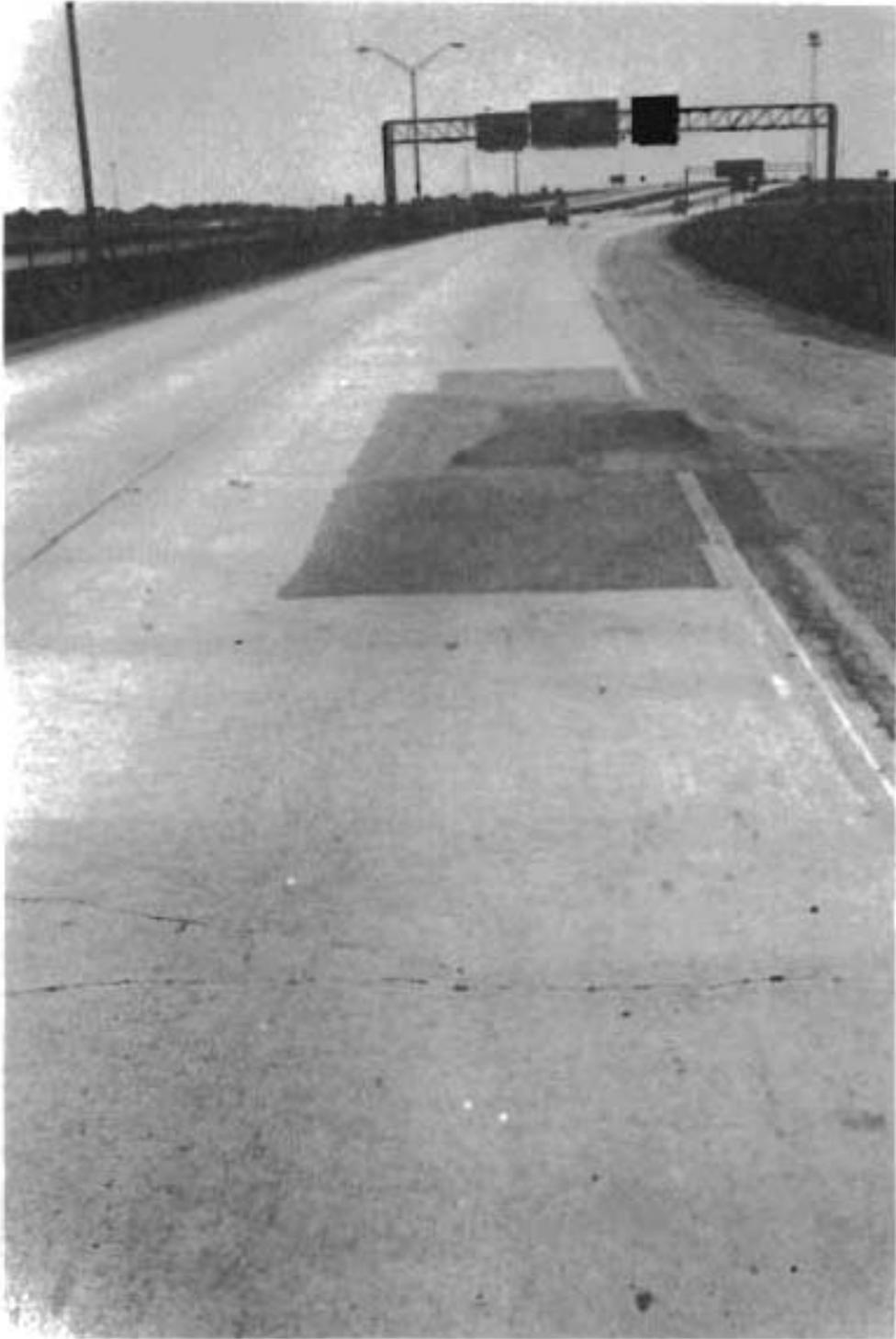
Fig 1.3. Multiple asphaltic patches; it appears there are five patches on top of each other in this location.
