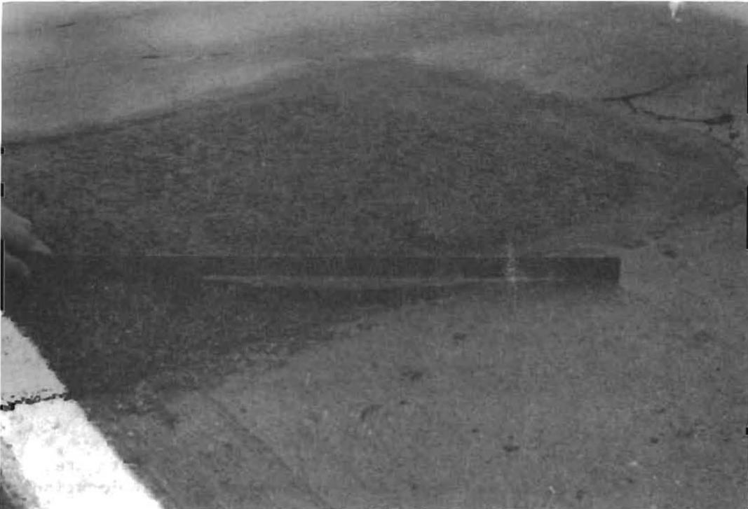
Fig 1.2. Asphaltic concrete patch exhibiting shoving.
