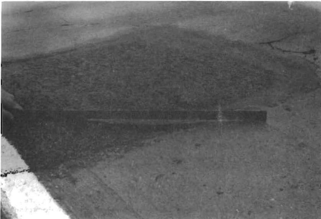
Fig 1.2. Asphaltic concrete patch exhibiting shoving.
