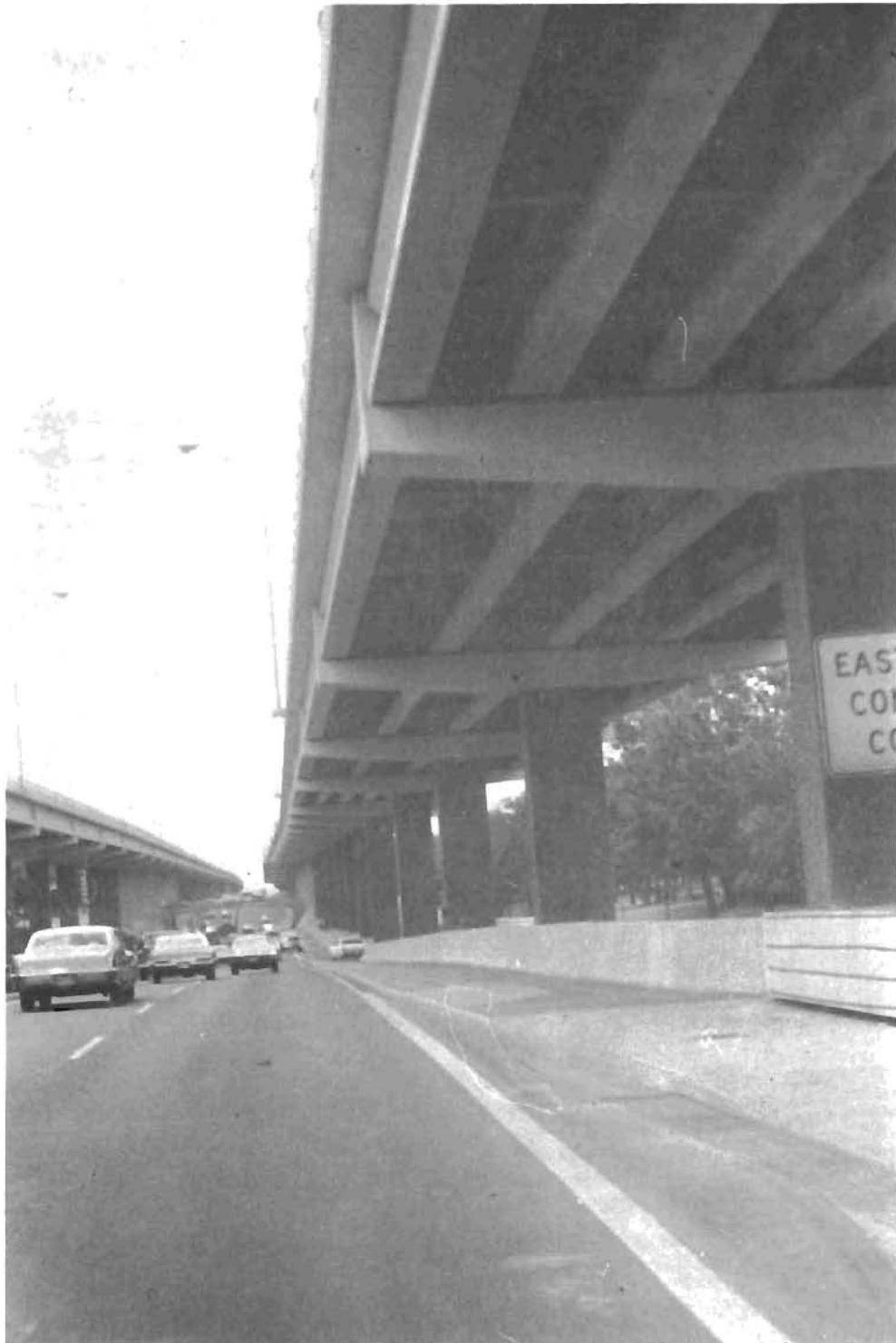
Fig. 1. Some inverted T-beam bent cap girders in place.
