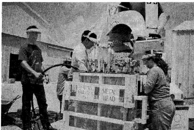
Figure 2.7 Placing concrete in column form
