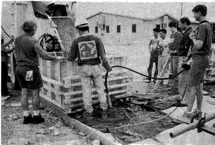
*Figure 2. 11 Placing concrete in footing form*
