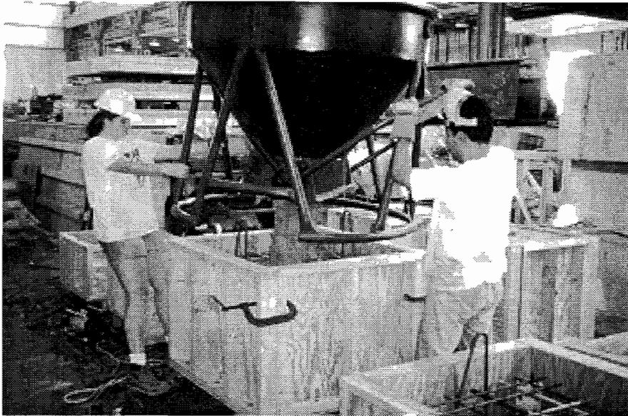
*Figure 4. 10* Placing concrete in specimen from overhead bucket
