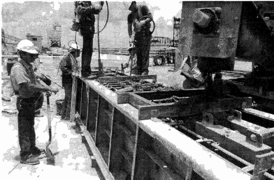
(b) Vibration of concrete in precast element
