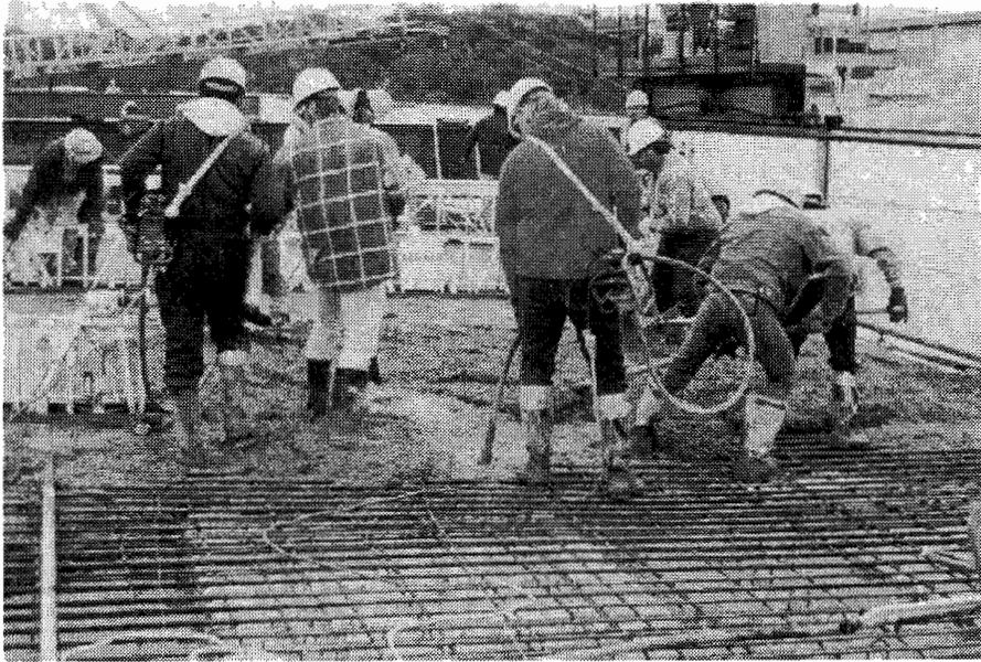
*Figure 1.3 Consolidation of concrete in bridge deck*
