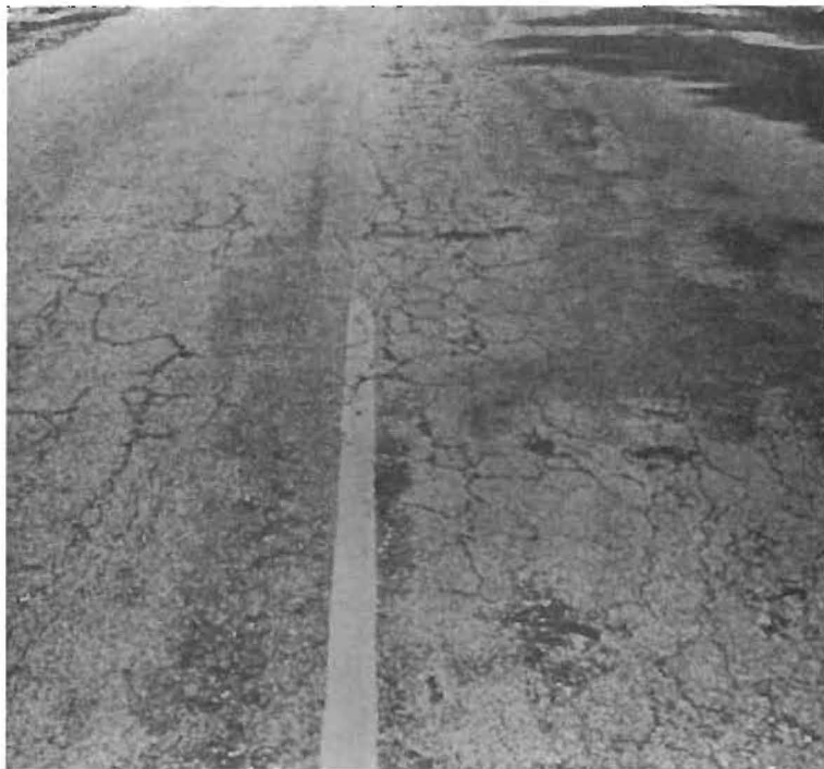
(d) Pavement failure due to insufficient bearing capacity.
