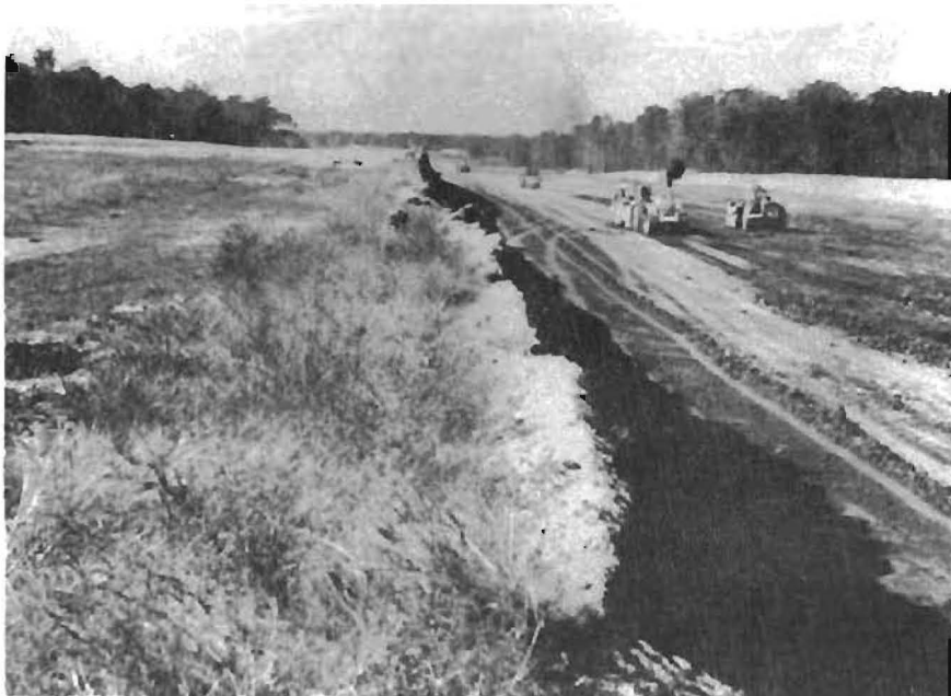
Fig 4.4. Clay cut with work in progress on westbound lane.
