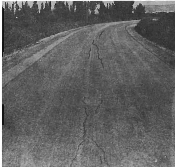
(b) Longitudinal cracks.
