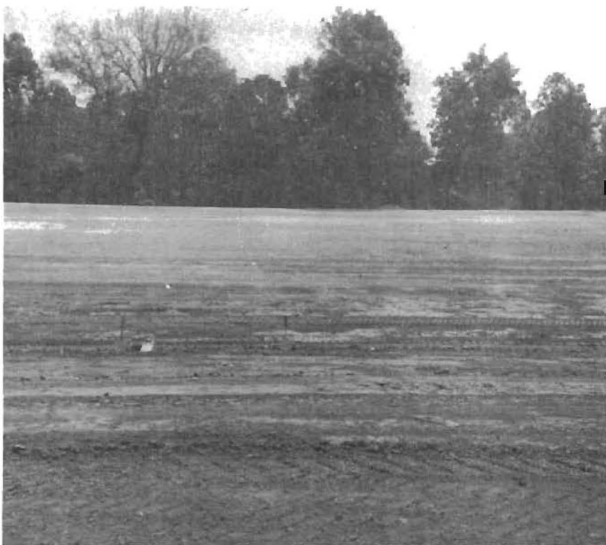
Fig 4.5. Completed clay cut. The three round paint cans mark locations of access tubes.
