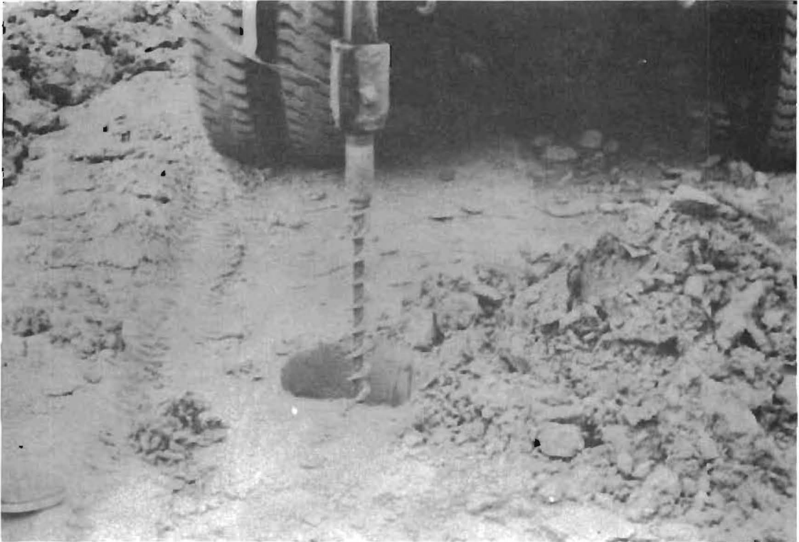
Fig 4.8. Drilling small hole for nuclear access tube.
