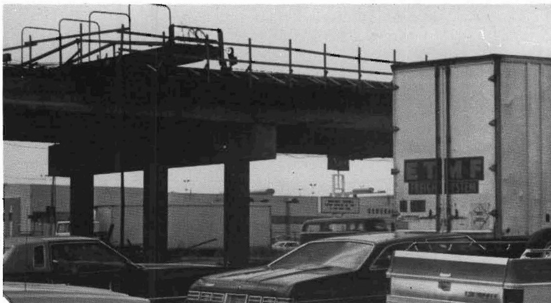
Construction at State Highway 360 and Abrams Street
