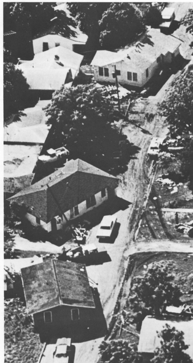
Floods of the same or larger magnitude as those that have occurred in the past can occur in the future.
