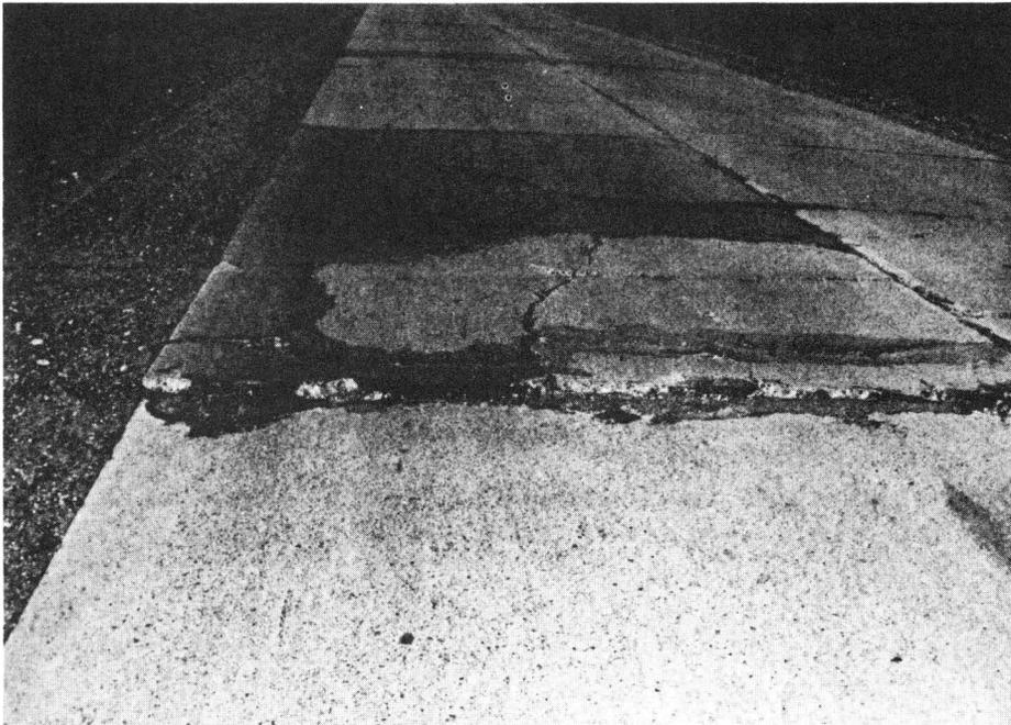
Figure 6.9 -- Shattered Slab
