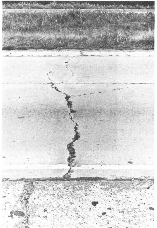
Figure 6.1 -- Failed Cracks
