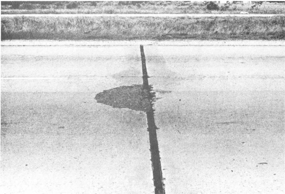
Figure 6.6 -- Failures (asphalt patches)
