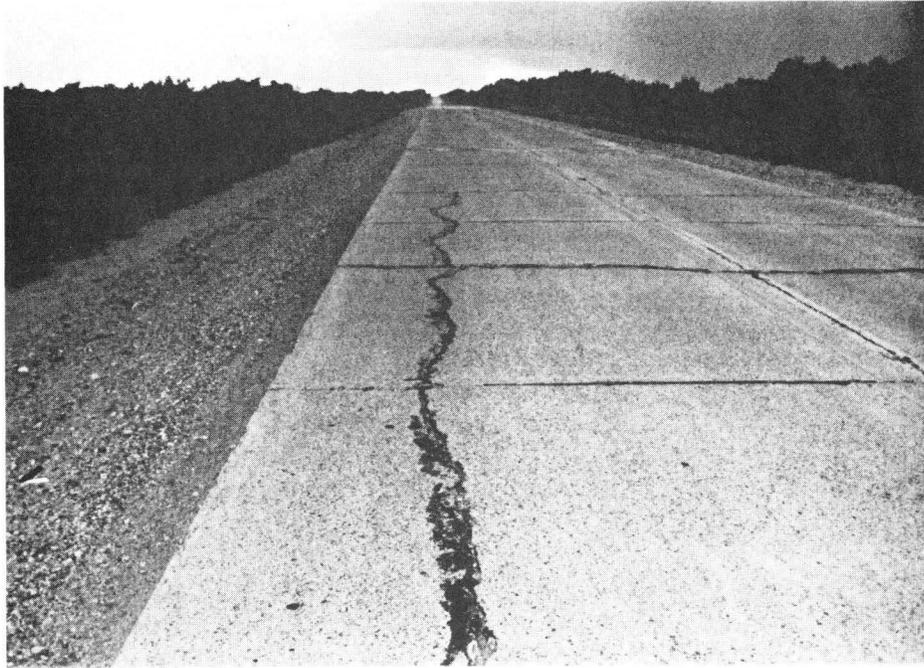
Figure 6.10 -- Slab with Longitudinal Crack
