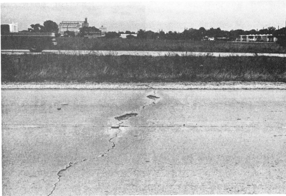
Figure 6.2 -- Failed Cracks (in far lane)
